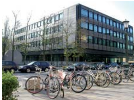
Figure 4-75 The Munich Re East building, Königinstrasse in Munich, Germany
