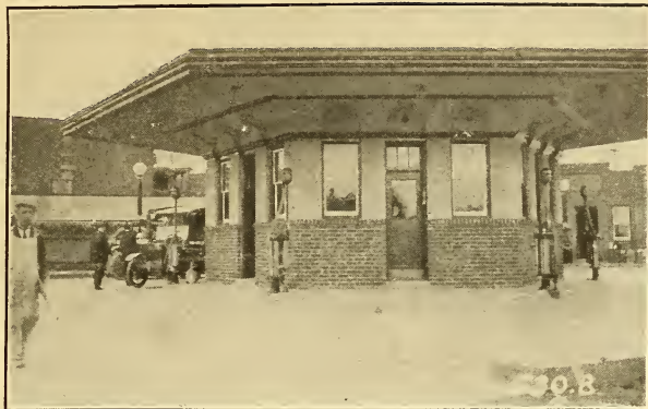
FIG. 1.—Example of large filling station, having 10 measuring pumps for gasoline and 4 for lubricating oil
