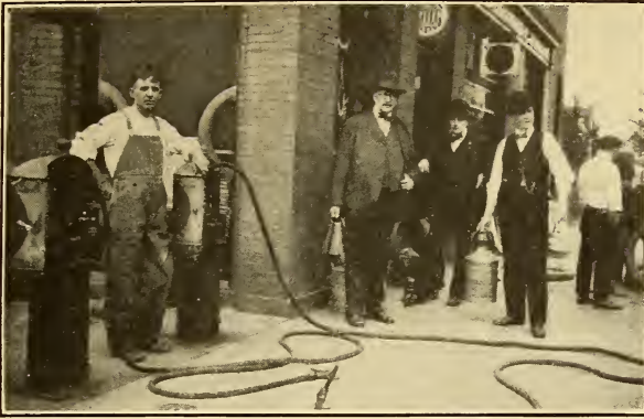
FIG. 15.—Excessively long hose due to pump being set back from curb. The practical impossibility of draining such hose into the purchaser's tank is obvious
