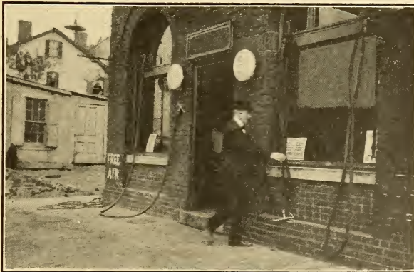
FIG. 17.—Delivery hose outside, pumps inside. Bad practice unless purchaser can clearly observe the operation of the pump from his position outside
