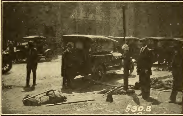
FIG. 16.—Showing hose connection at curb level, making it impossible to secure complete or uniform drainage in service
