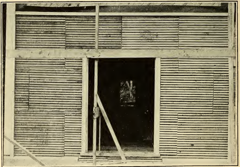
FIG. 32.—"Bishopric Board" on panel No. 51, left half creosoted lath, right half uncreosoted lath. Same construction on panel No. 52
