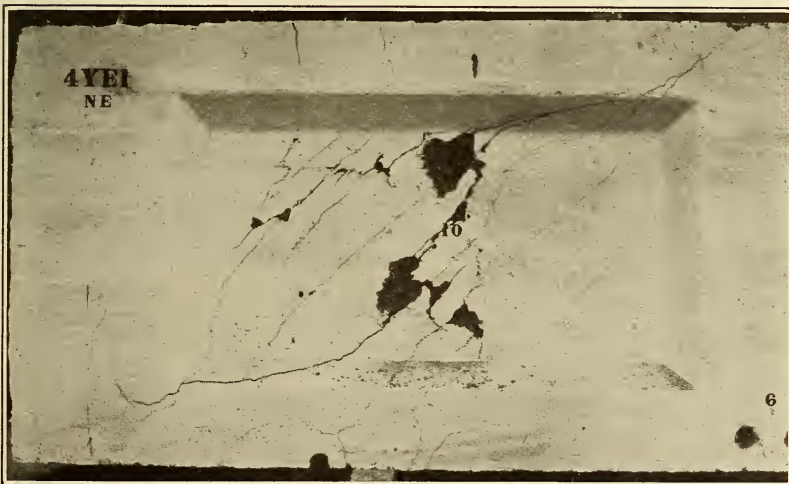
FIG. 22.— Failure of beam 4YE1 by vertical shear combined with diagonal compression
