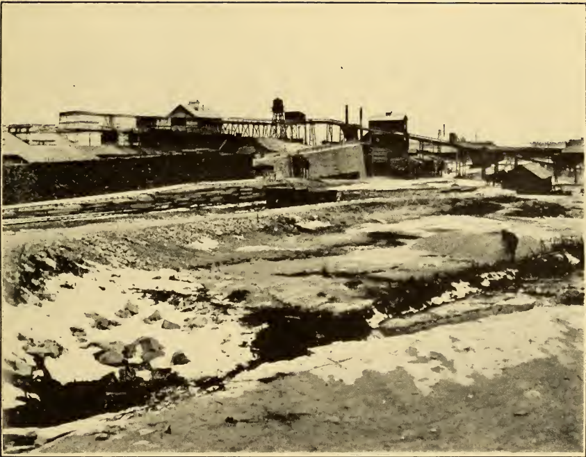
Fig. 30.— Manistique Plant of the White Marble Lime Co.
