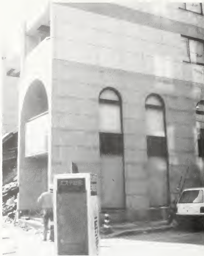
Figure 3.5.35 Seven-story steel frame SAGA Building - Flower Road in Kobe.
