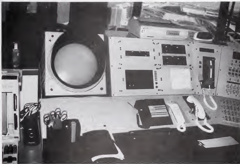
Figure 4.4.14 Supervisor control position located in center of control tower Cab.
