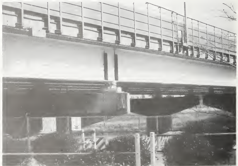
Figure 4.2.9 General view of Mukogawa Bridge, Meishin Expressway.
