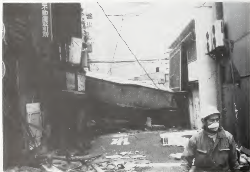
Figure 6.2.24 Road blocked by collapsed structure.
