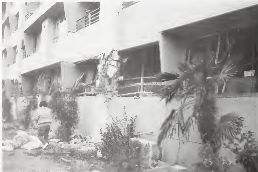
Figure 3.4.11 Short column effects - Fukae Mitsuku Housing Project.
