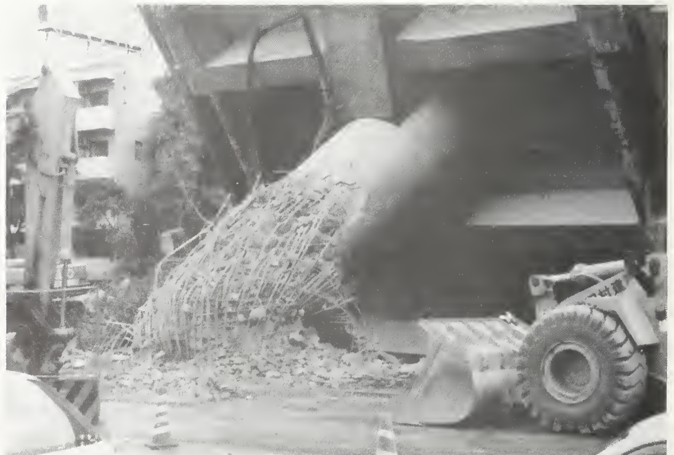
Figure 4.2.16 Higashi-Nada Viaduct, Pier 134.
