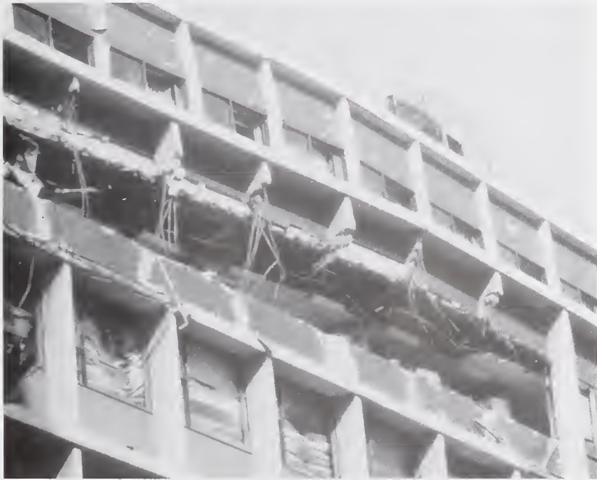
Figure 3.4.22 Upper story collapse - Downtown Kobe.
