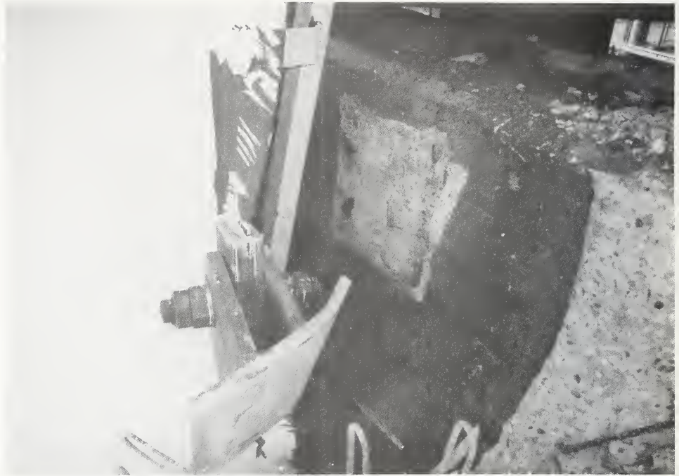
Figure 4.2.11 Damaged restrainer at Abutment A1, Mukogawa Bridge, showing failure of anchor bolts and distortion of web of main girder.
