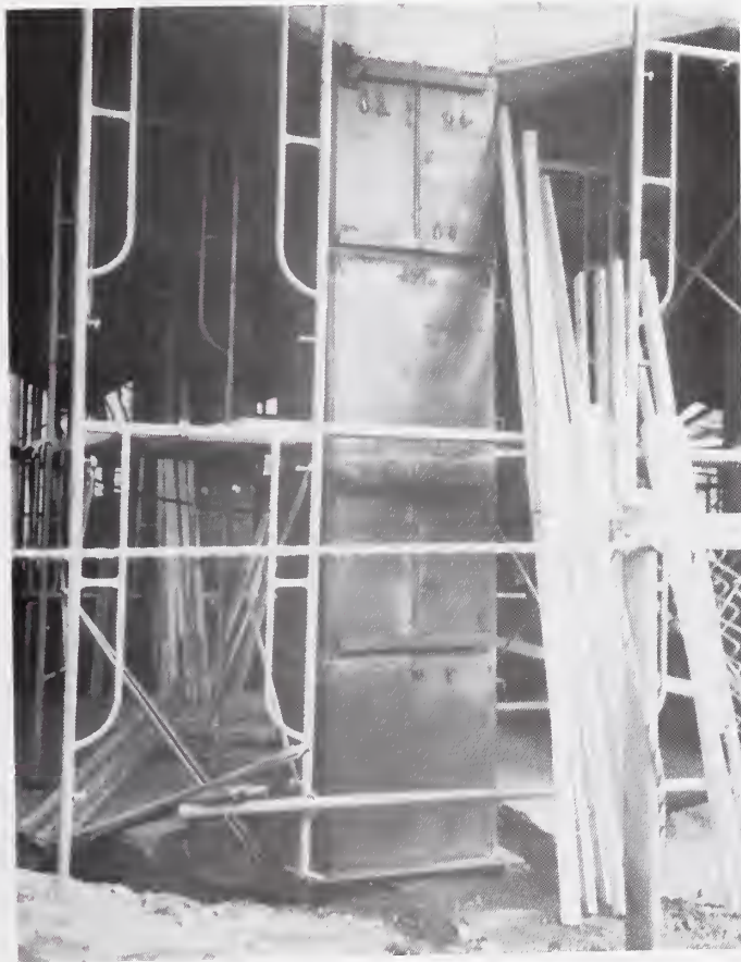
Figure 4.3.8 Jacketed column - JR Main Line.
