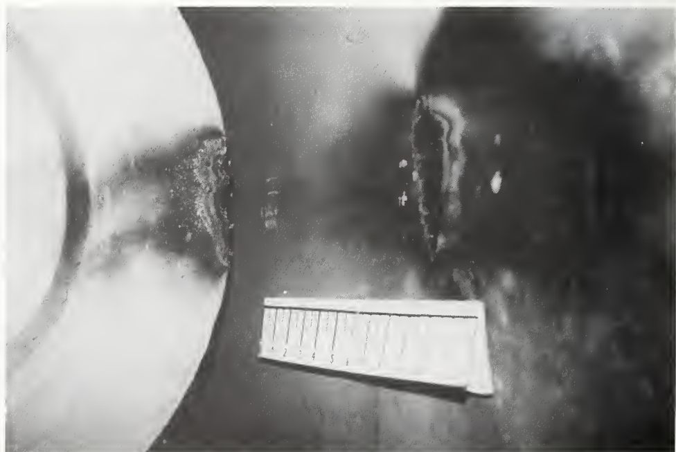
Figure 5.4.36 Movement of transformer damaged cabinet and shorted transformer case the tertiary output.
