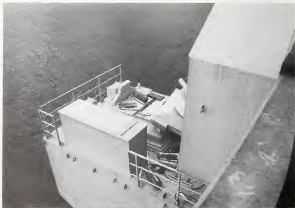
Damaged expansion bearing and lateral offset of west face of South Pier, Rokko Island Bridge.
