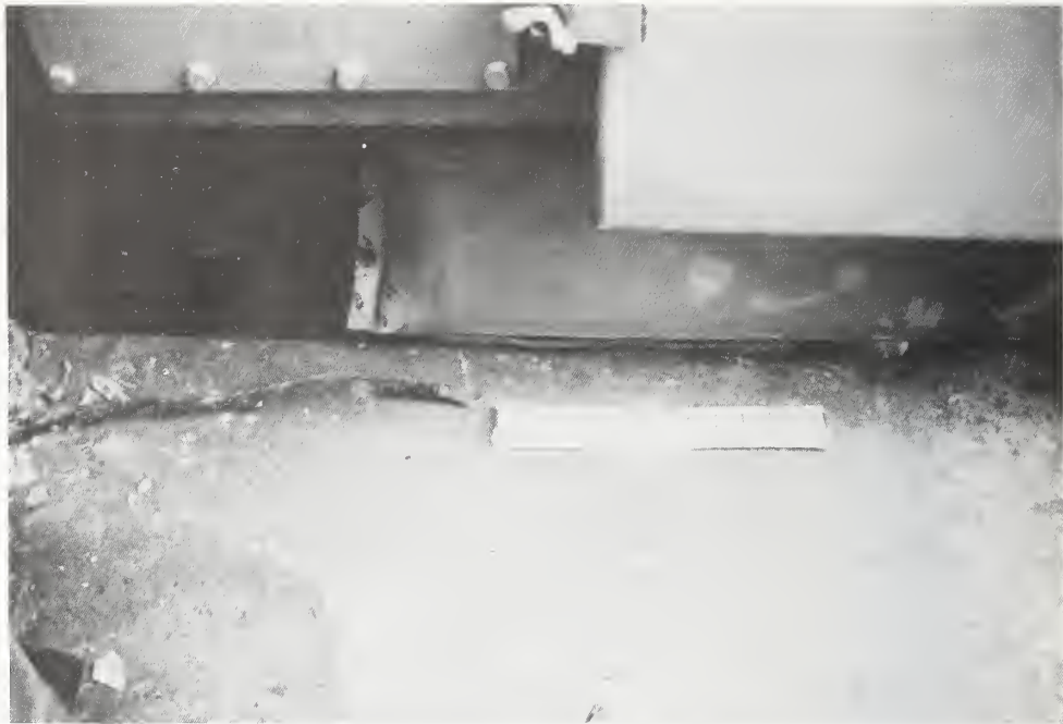
Figure 5.4.35 Transformer control cables were almost sheared off due to movement of the transformer.
