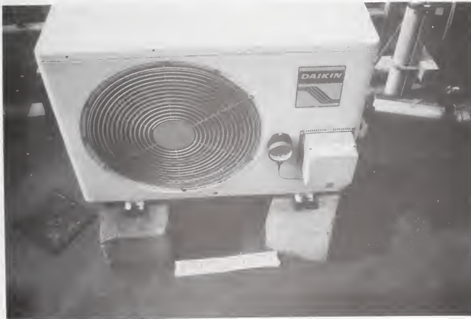
Figure 4.4.23 Heat exchanger on roof near control tower cab is rare example of poorly anchored equipment.
