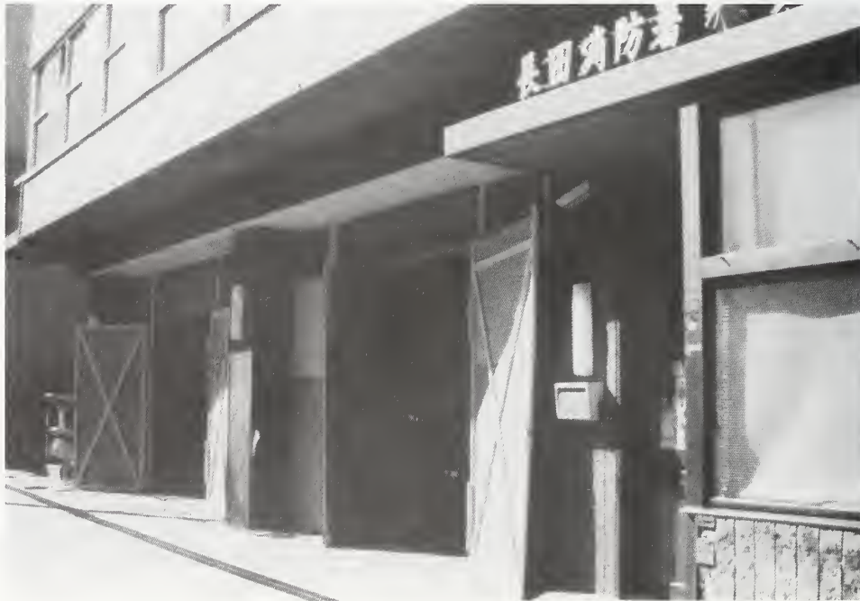
Figure 6.2.28 Fire station damaged by the earthquake.
