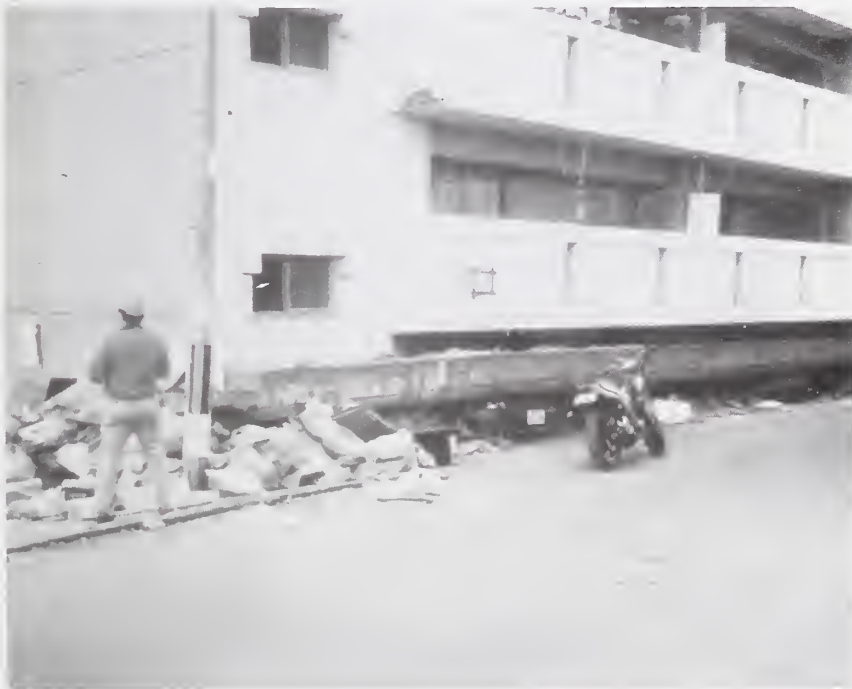
Figure 3.4.5 Failed ground floor shear wall - apartment building.
