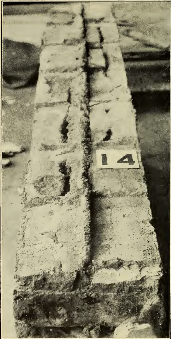
FIGURE 7.— The mortar bed in a wall of series 1 Wall 14, an 8-inch solid wall built of Chicago brick, laid in cement mortar.
