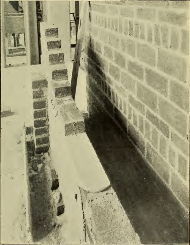
FIGURE 12.— Carefully leveled horizontal mortar beds in the walls of series 2 518—7
