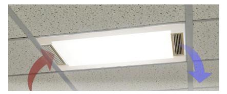
Fig. 14. Ceiling-mounted UV-C air purifier [28].
