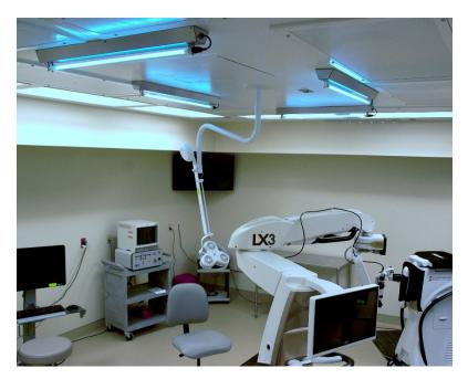
Fig. 11. Ceiling-mounted room disinfection fixtures [25].
