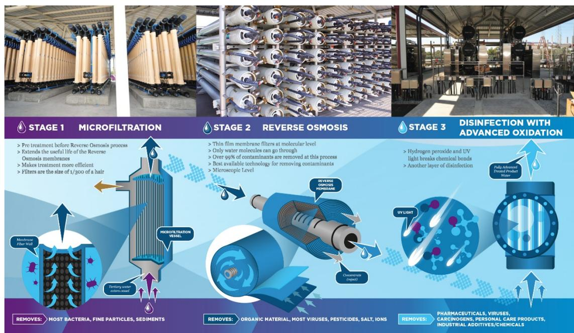
**Fig. 7.** Advanced water treatment process at the Water Replenishment District of Southern California (WRD) Leo J. Vander Lans Water (LVL) Treatment Facility [57]. Stage 3 includes the use of UV radiation for the disinfection of microorganisms and other components that are broken down due to advanced oxidation processes catalyzed by photolysis reactions of water with UV radiation. Figure credit: WRD LVL.
