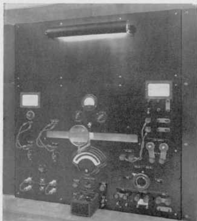
FIGURE 5. Instrument testing panel, including Lindeck element.
