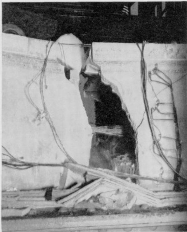
FIGURE 23. Fracture at midspan of the girder tested at 0° F.
