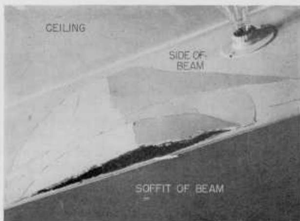
FIGURE 14. Plaster failure involving the expansion of about 0.5 percent in the white coat along the side of a concrete beam.
