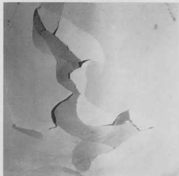
FIGURE 2. Bulging of white coat on a side wall, involving separation of the finish (or white) coat from the sanded gypsum base coat within an area of about 1 sq yd.
