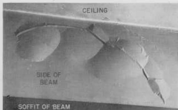
FIGURE 1. Bulges in white coat along the side of a concrete beam, caused by the expansion attending the slow hydration of free MgO present in the hydrated lime used in preparing the white coat.
