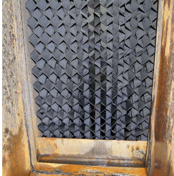
Figure 5. Vertical metal matrix assembly used in first stage of the wet scrubbing system.
