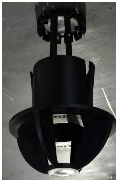
Figure 4. One of seven spray nozzles used to scrub soot in the first stage of the scrubbing assembly.
