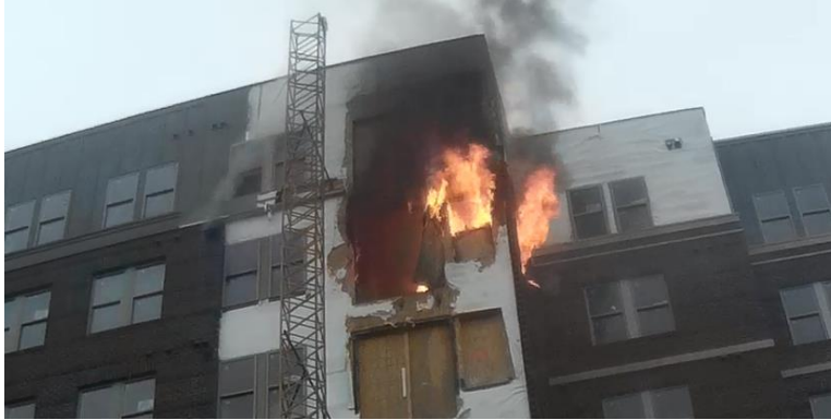
Figure 2. Still image from approximately 9:41 AM showing severe damage to construction doors on exterior of 6th floor apartment and flames extending out of the southeastern and eastern windows from the 6th floor apartment [2:09 SID Helmet Cam].
