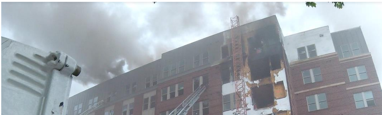
Figure 8. Smoke venting from the roof-level passive ventilators at approximately 10:18 AM [4:00 We Need 10ft Hooks (V5)]
