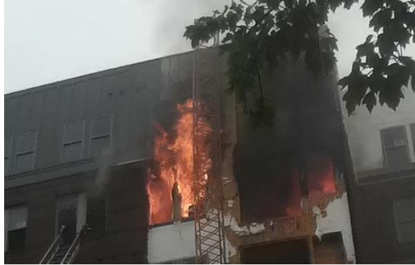
Figure 5. Still image from approximately 9:49 AM showing flames extending out of the 6 th floor apartment bedroom window openings with apparent re-ignition in the original fire room [10:11 SID Helmet Cam].
