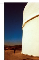
Buckle in the 2- million gallon Sesnon Tank where steel plate thickness changed from 9/16-inch to 7/16-inch – LADWP photo
