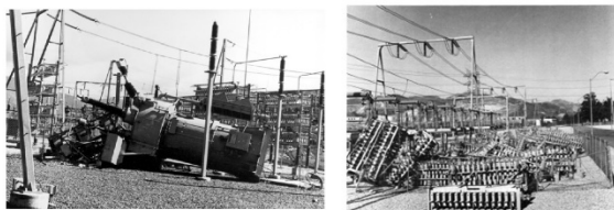
Damaged Power Equipment at Sylmar Switching Station – LADWP photos
