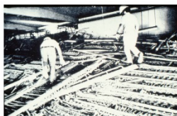
Electro-mechanical equipment collapsed
