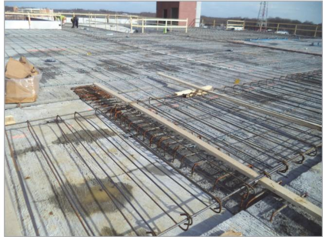
**Figure 9-1.** Reinforcement placement in progress for topping slab diaphragm with step in floor elevation.
