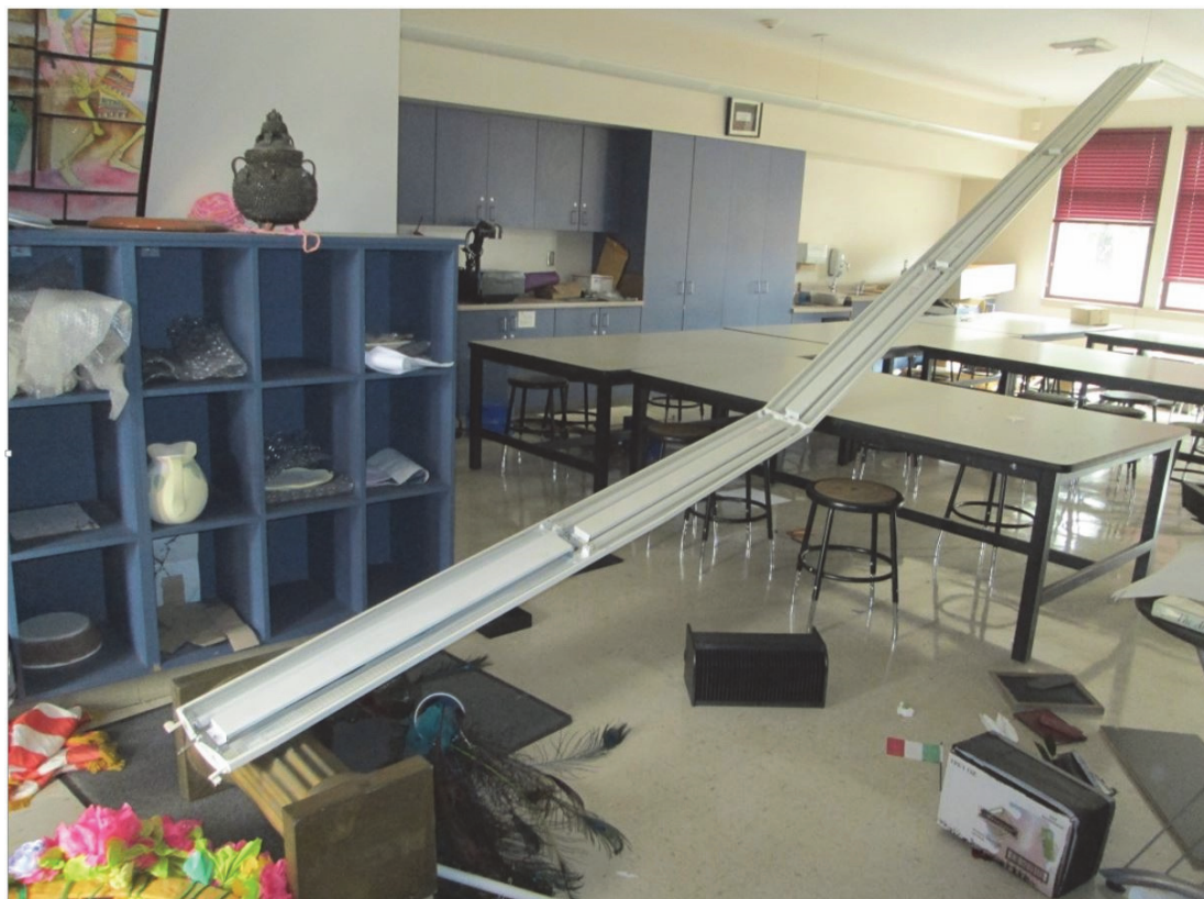
Figure A-4 Suspended light fixture is dislodged and falls.
