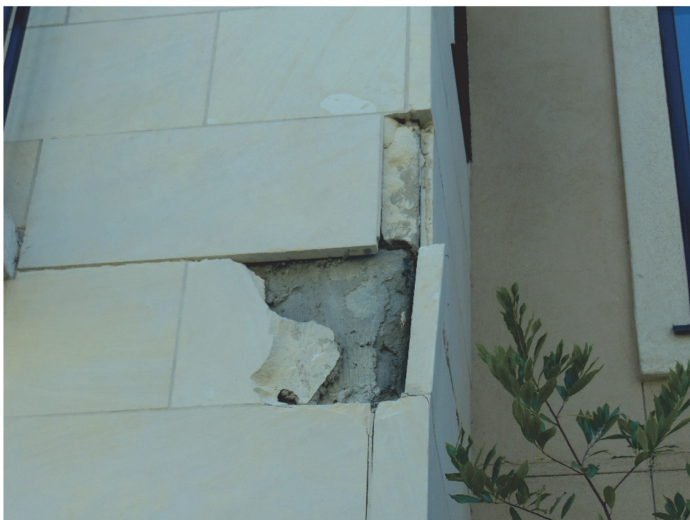
Figure 2-6 Adhered veneer damaged during the 2014 South Napa earthquake (FEMA, 2015a).
