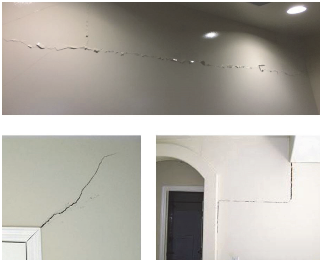
Figure A-3 Gypsum wallboard cracks.
