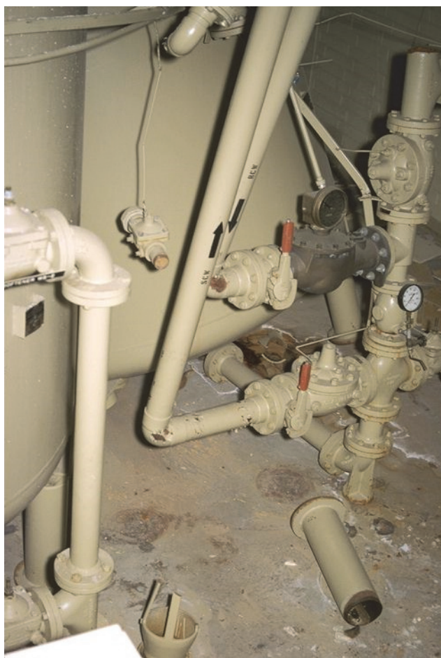
Figure 2-2 Broken piping in the new power house for the Olive View Hospital, 1971 San Fernando earthquake (NISEE, 2016b).
