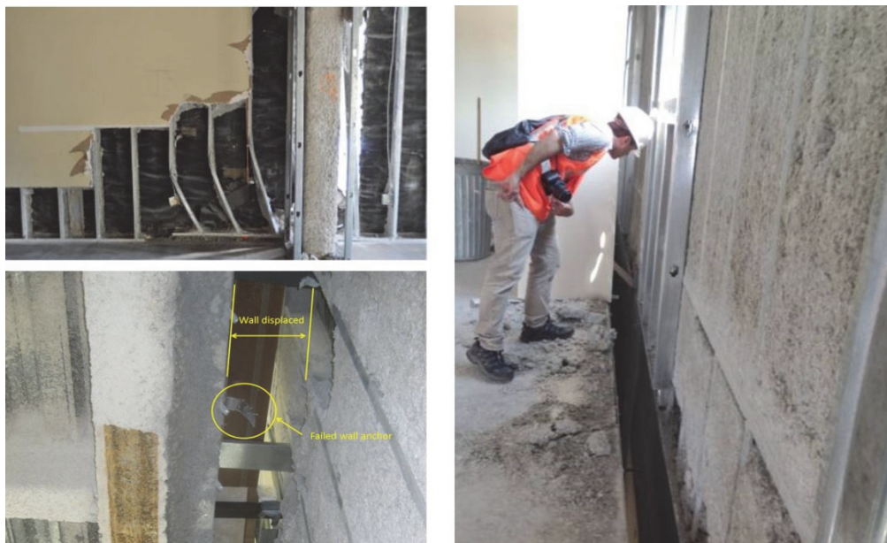
Figure A-1 Lightweight exterior cladding is damaged and requires replacement, but there is no safety concern due to falling panels.
