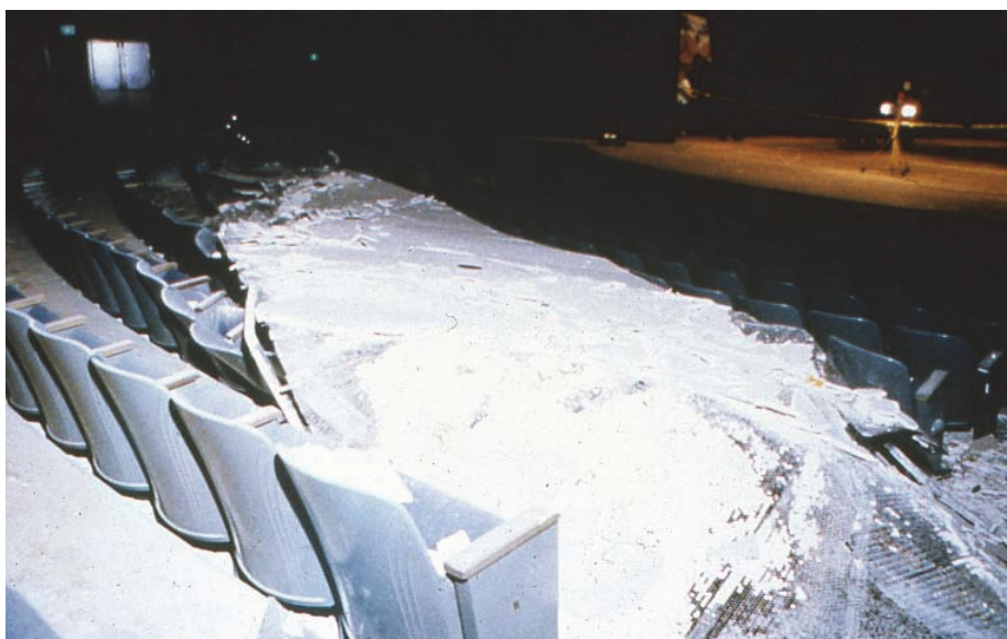
Figure 2-4 Collapsed heavy ceiling in the Geary Theater, San Francisco, California, 1989 Loma Prieta earthquake (NISEE, 2016c).
