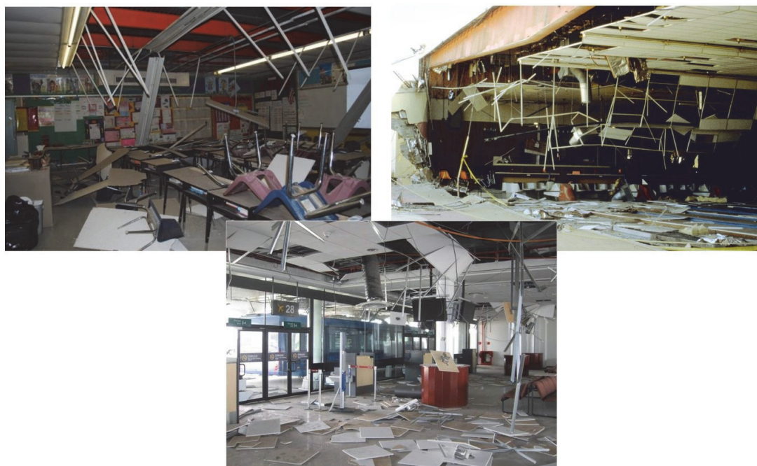
Figure A-8 Acoustic tile ceiling grid is damaged and requires replacement.
