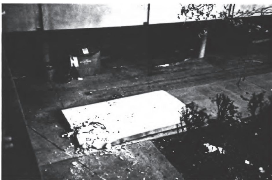
Figure 2-3 Fallen precast concrete panel at the California State University Los Angeles parking structure, 1987 Whittier Narrows earthquake (Çelebi et al., 1987).
