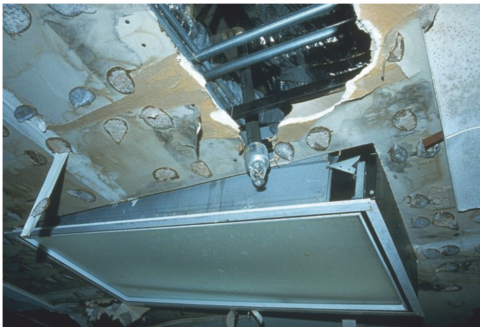
Figure 2-5 Fractured sprinkler line and dislodged light fixture in the Olive View Medical Center, 1994 Northridge earthquake (NISEE, 2016d).
