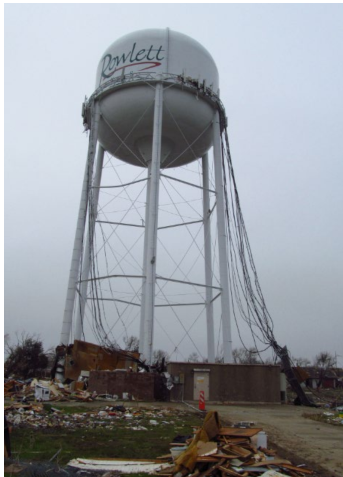
Figure 6. Water tank of the city of Rowlett, Texas, showing significant structural damage (note the bent horizontal braces) after being struck by a tornado in December 2015.
