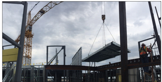
Figure 3-1. Example of panelized floor being erected.
