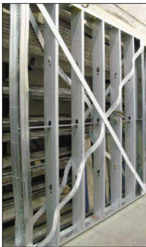
(d) Strap-braced wall after testing, showing yielding in strap (adapted from Comeau 2008 Figure 2.23)
