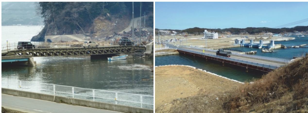
Figure 6-1 Temporary bridge restoring coastal highway in Minamisanriku, Japan (N 38.673519, E 141.443135) (left) (one month after March 11, 2011 tsunami); and more substantial replacement bridge built 4 months later (right). (Photos courtesy of Ian Robertson).
