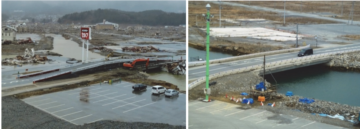
Figure 6-2 Temporary bridge restoring coastal highway in Rikuzentakata, Japan (N 39.009206, E 141.630195) (left) (one month after March 11, 2011 tsunami), and bridge repaired within one year (right). (Photos courtesy of Ian Robertson).
