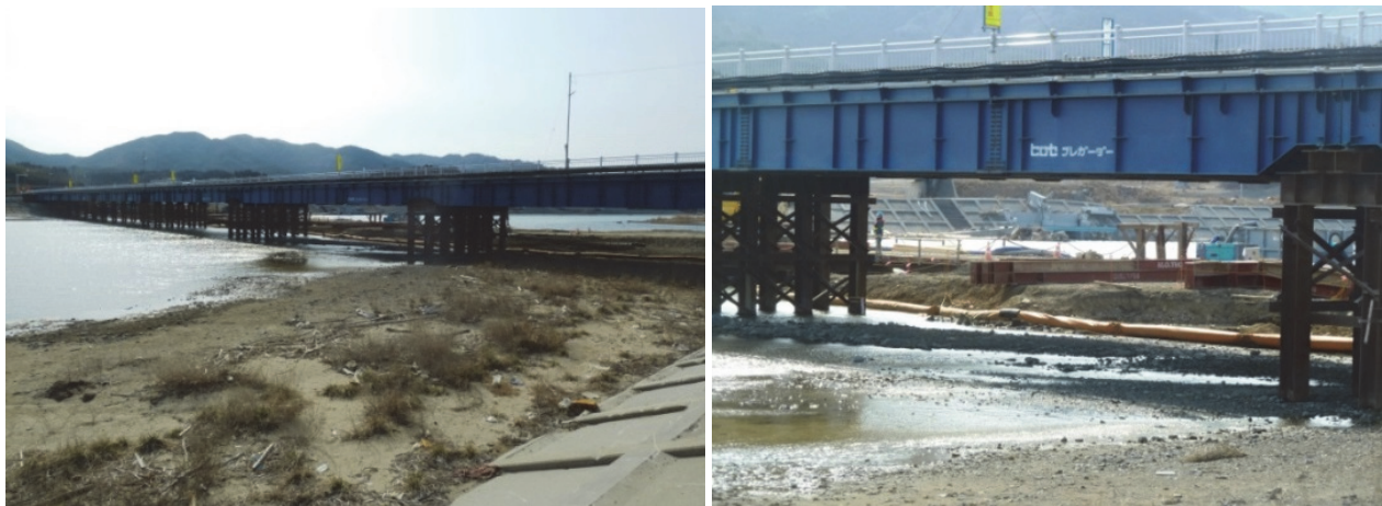
Figure 6-3 Temporary steel girder bridge over river in Koizumi, Japan (N: 38.67933, E: 141.50787), just North of Utatsu, Japan, completed 107 days after the March 11, 2011 tsunami. (Photos courtesy of Ian Robertson).
