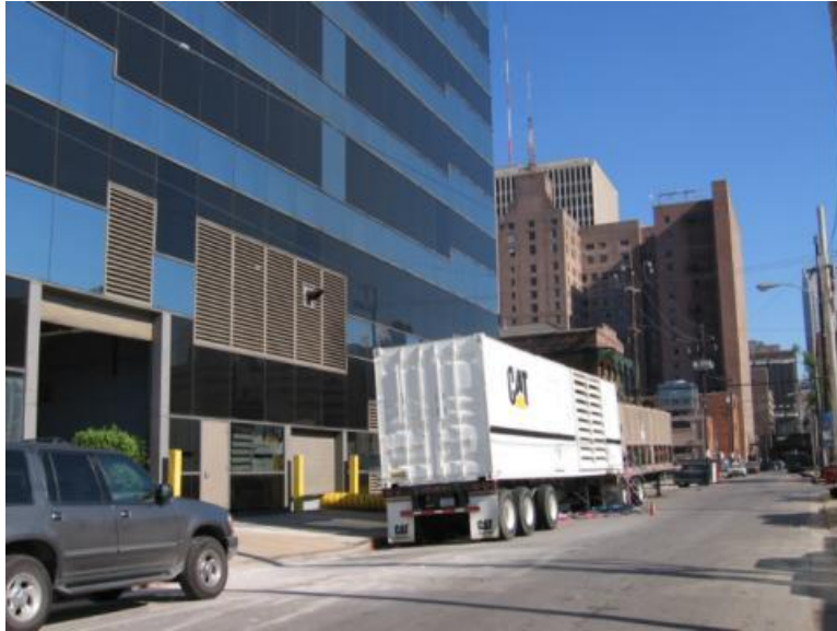
Figure 20. A portable generator in front of Tulane University School of Medicine after Hurricane Katrina. The building is equipped with a permanent generator that was not operational.
