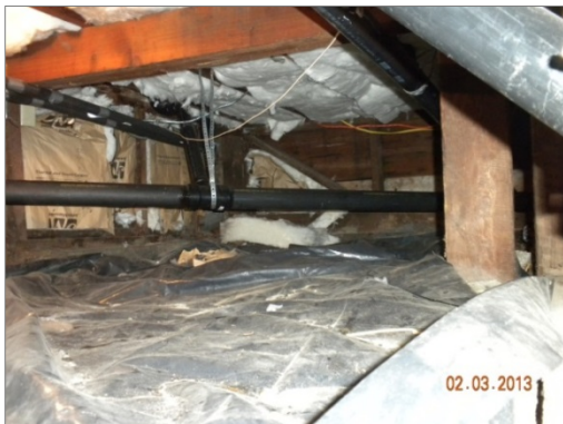
Insulation in crawlspace attached to the conditioned basement. The crawl was vented but had a poorly defined pressure boundary between the crawl and the basement, which made a large contribution to the overall house air leakage. Some wall and floor insulation was displaced and ducts were un-insulated and poorly sealed.
