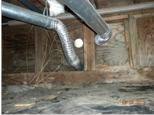
Dryer vent disconnect from outside in crawl
