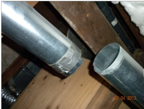
Disconnected dryer vent in crawlspace
