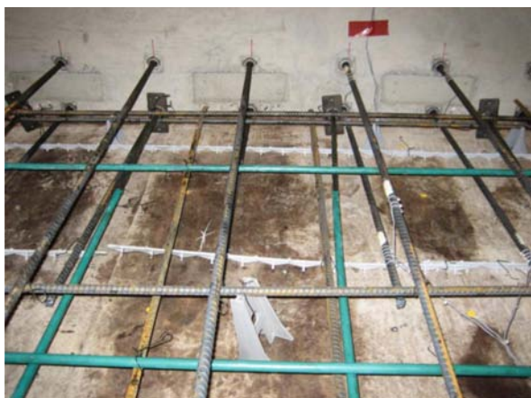
Figure 9-4 – Form savers for dowel anchorage.
