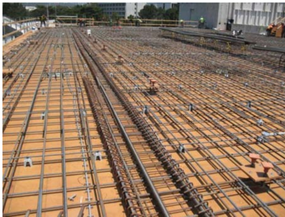
Figure 9-2 – A long collector with confinement reinforcement.
