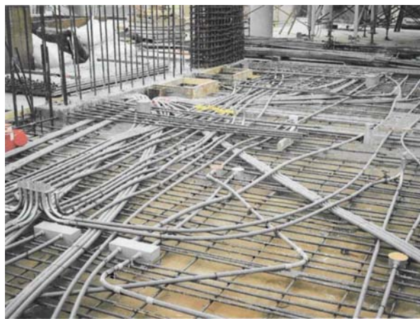
Figure 9-5 – Embedded conduit.
