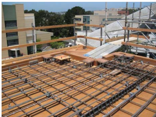
Figure 9-3 – Confinement of a collector.
