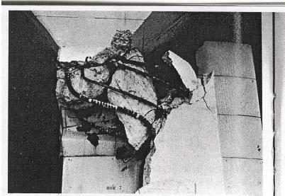
Figure 2.7 Large Lateral Deformations and Failure of Columns at Sixth Floor of Military Personnel Records Center
