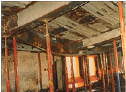
Figure 2.9 One Meridian Plaza Interior Fire Damage
