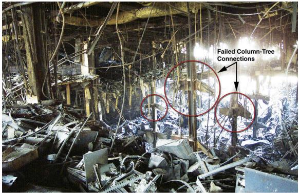
Figure 2.1d Partial Connection and Floor Failures in WTC 5
