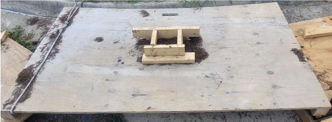
Figure 7. A photograph of a plywood tree platform prior to mounting of the tree.
