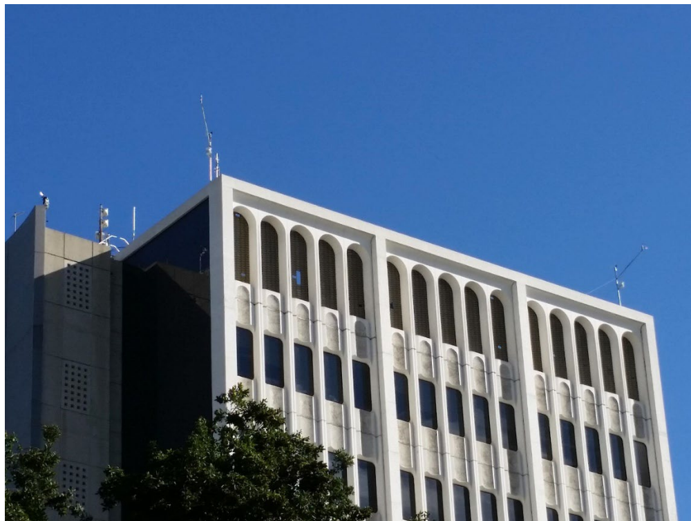
Figure 20. Air inlets and weather stations at the four corners of the roof of Caltech Hall on the Caltech campus in Pasadena, Calif. (Photo courtesy of Earth Networks, Inc.)
