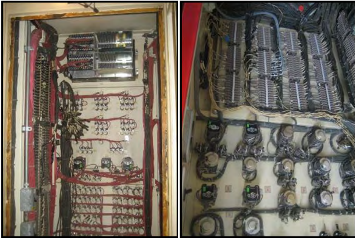
Fig. 1. Photographs of electrical enclosures typically found near the main control room in a Nuclear Power Plant.
