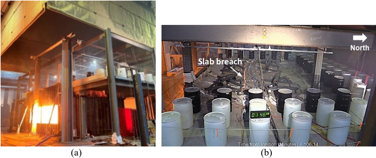
Fig. 1. Test #1 (a) compartment fire test in the south middle bay of the two-story building under 20 MW exhaust hood; (b) top of the composite floor developing slab breach at 106 min after burner ignition.
