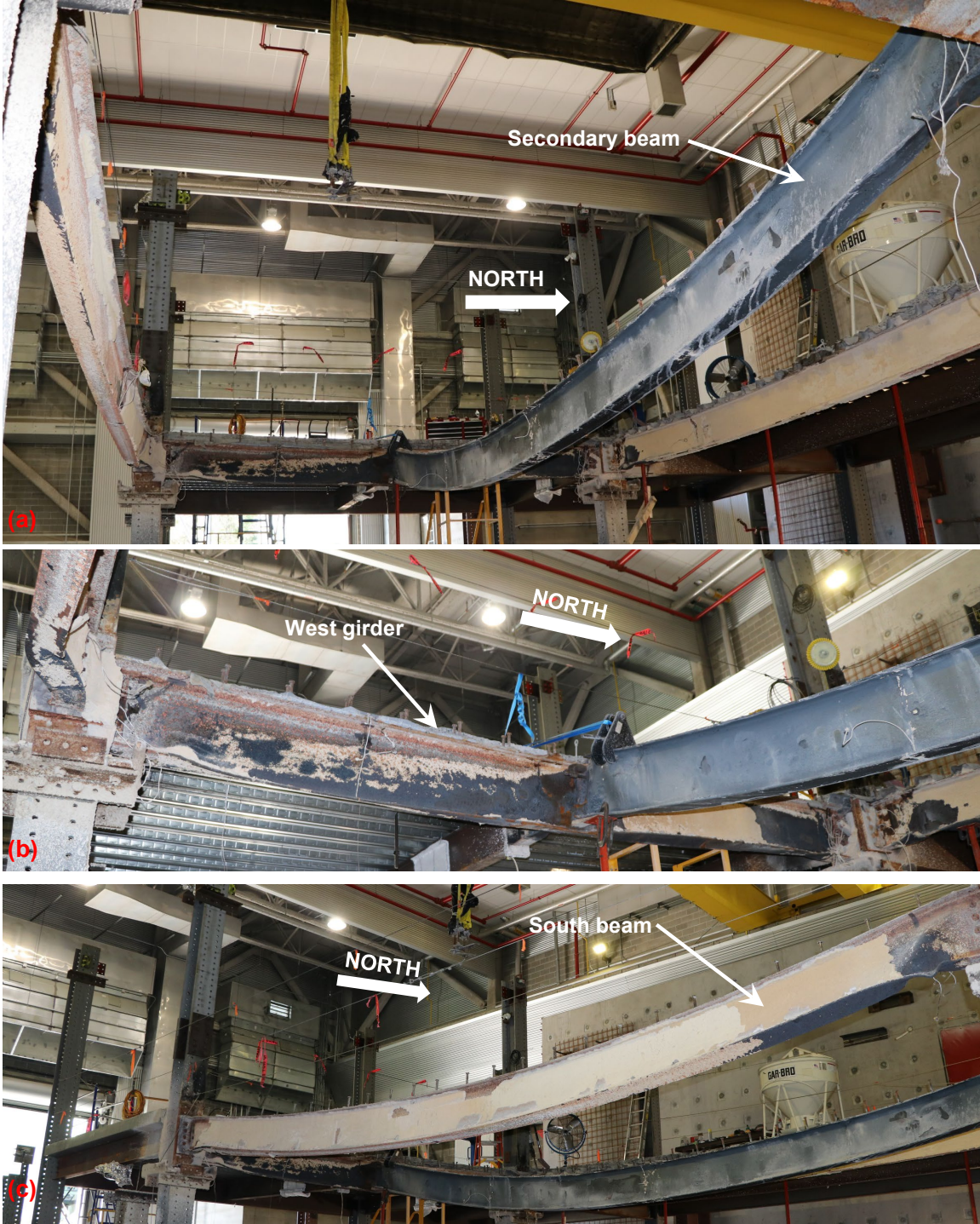
Fig. 41. Post-test photographs of the test bay beams after steel deck removal.
