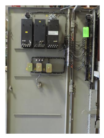
Fig. 8. Photo of combustible component loading in the secondary enclosure
