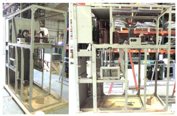
Fig. 4. Type M-36 Metal Clad Enclosure (note: bus bar and breaker not shown)
