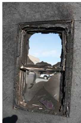
Fig. 49. Photographs showing window damage for different exposures.
