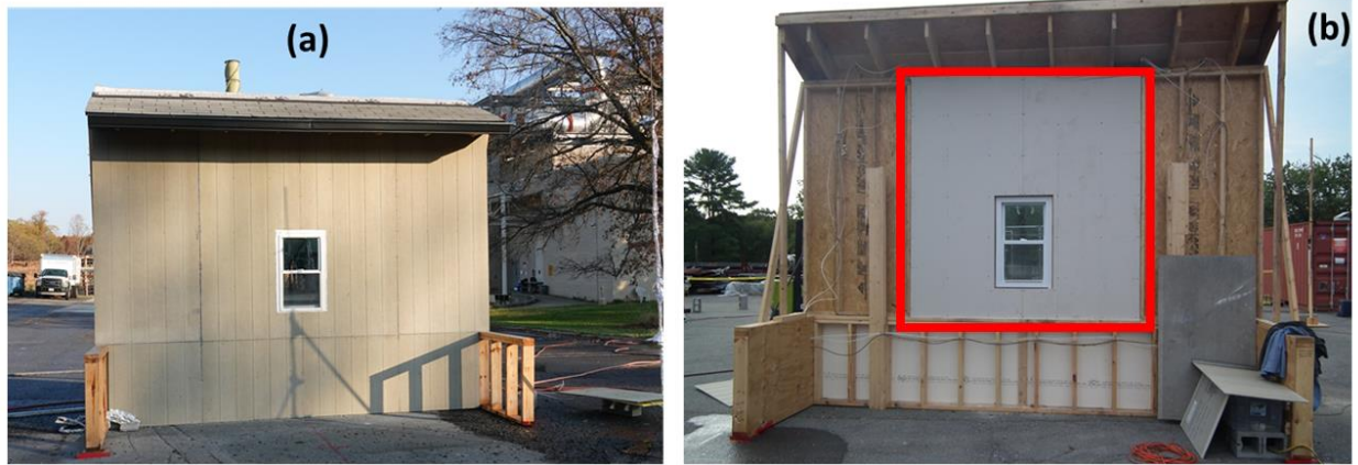
Fig. 20. Photograph showing (a) front view and (b) rear view of the target structure. The area highlighted by the red outline denotes the portion of the replaceable complete wall assembly.
