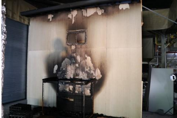
Fig. 47. Photograph showing spalling of exterior layer (cement board) in indoor test 1B-WCI0-0.
