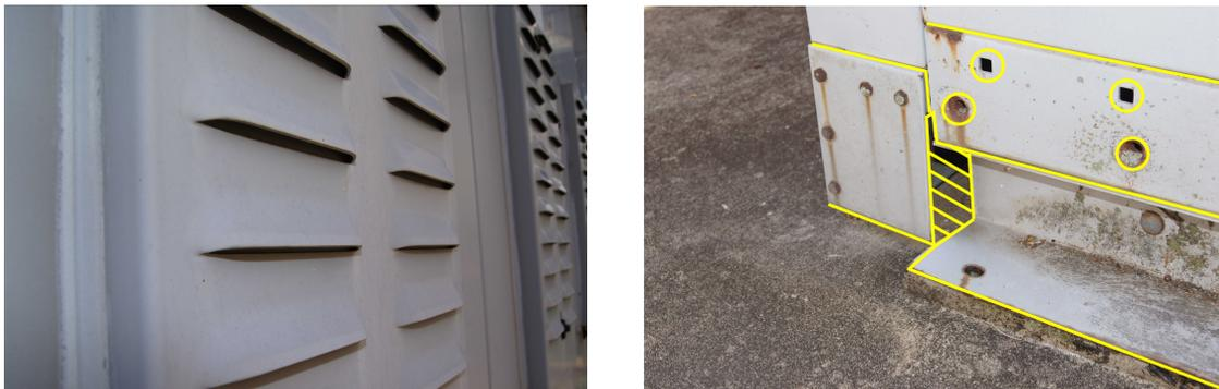
**Fig. 10.** Louvers and miscellaneous leakage paths (yellow lines).
