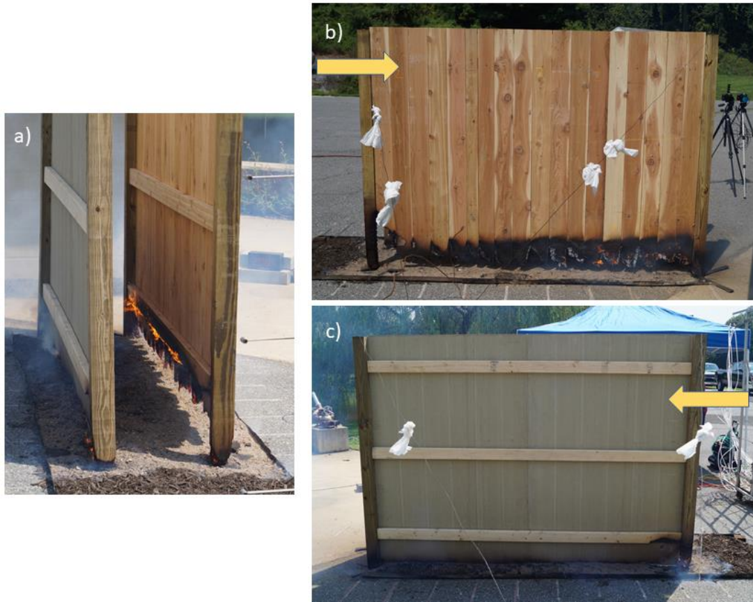
Fig. 133. Cement board (noncombustible) parallel to WRC privacy fence with 46 cm (18 in) spacing, near end of experiment, in camera views from a) near the fan, b) right side, and c) left side [Test C-15]. Arrows indicate wind direction.
