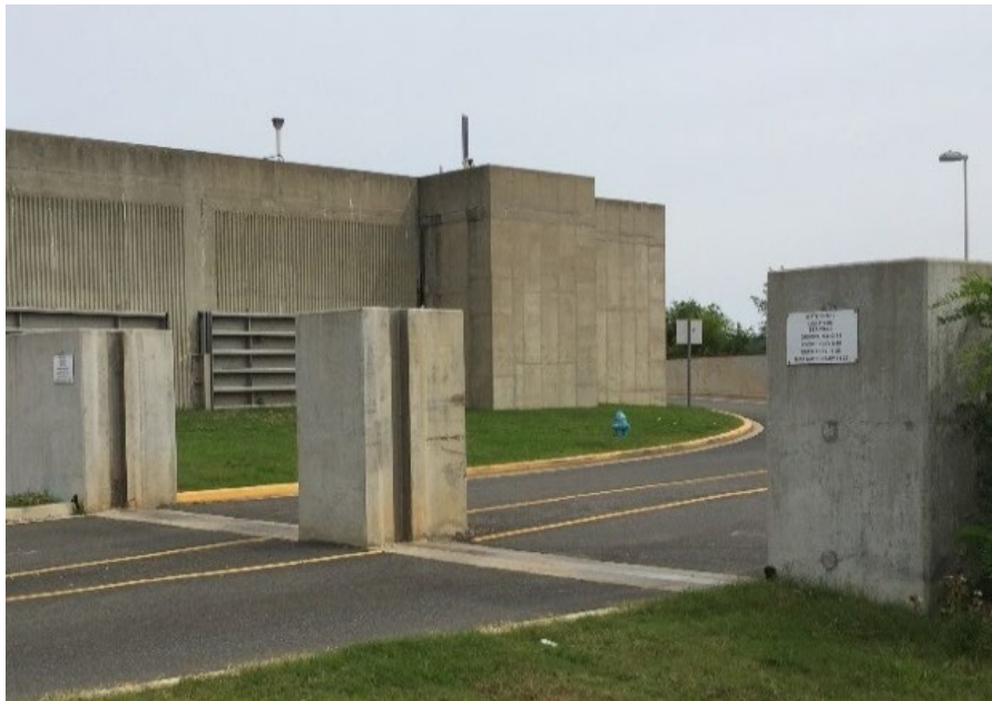
Figure 3-5: Flood Protection Barrier with Removable Gates Across Roadway
