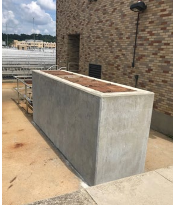
3.2.5.2 Figure 3-6: Raised Gate Access Above Conduit Flood Surge Elevation Stormwater Best Practices
