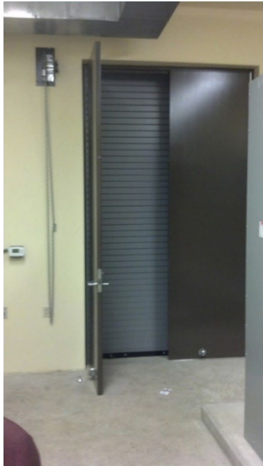
Figure 3-3: Hurricane Door Outside Double Door to Electric power Building / Tank Fill Guidelines
