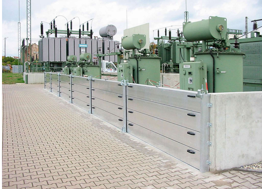
Figure 3-4: Barriers for Flood Protection Where Assets Cannot Be Raised
