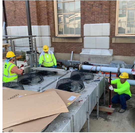
Figure 3-2: Example of Raising Vulnerable Infrastructure Above Floodplain Elevation
