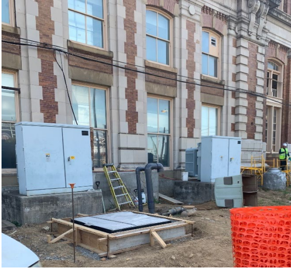
Figure 3-2: Example of Raising Vulnerable Infrastructure Above Floodplain Elevation
