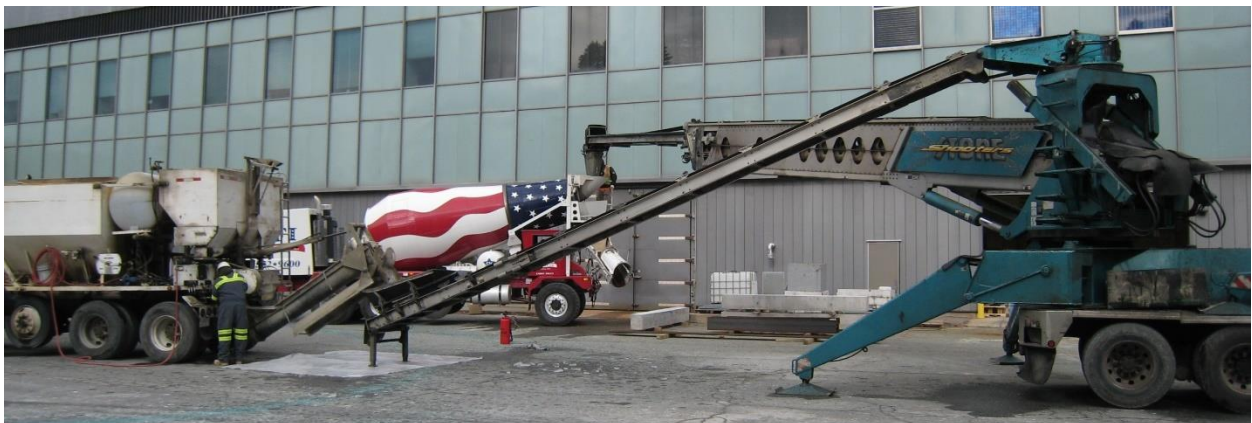
Figure 2.5. Loading the volumetric truck contents to a concrete mixer truck via a conveyor belt (telebelt)
