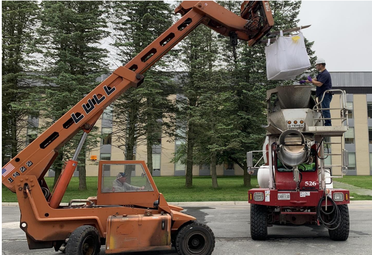
Figure 2.7. Loading of aggregates into concrete mixer truck
