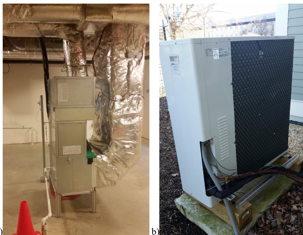
Figure 5: SDHV system indoor and outdoor units at the NZERTF, a) indoor air handler and b) outdoor unit
