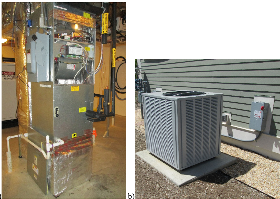
Figure 4: CDHP system indoor and outdoor units at the NZERTF, a) indoor air handler and b) outdoor unit
