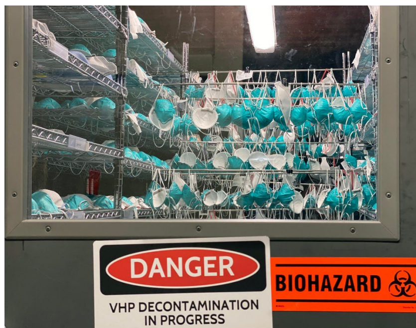
Figure 1: Battelle Memorial Institute VHP masks decontamination system. (Photo used with permission of John Clay).
