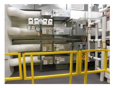
Fig. 10. Picture of the VAVs. The AHUs are to the left and the ZSs are to the right.
