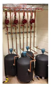
Fig. 13. The black tanks hold water for the thermal mass coils in the zone simulators. Above the tanks are the red circulating pumps that move the water through the TMCs. The flow rate is determined by manually setting a valve.
