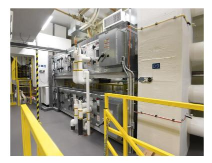
Fig. 8. AHU2 (top) and AHU1 (bottom). The OAU is on the upper mezzanine at the far left of the picture and the VAVs, not shown, are to the right.
