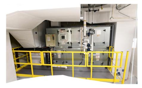
Fig. 6. Picture of the OAU. Air is drawn in from the lower left, exits the OAU on the upper left of the unit, and goes to the AHUs at the right (not shown).
