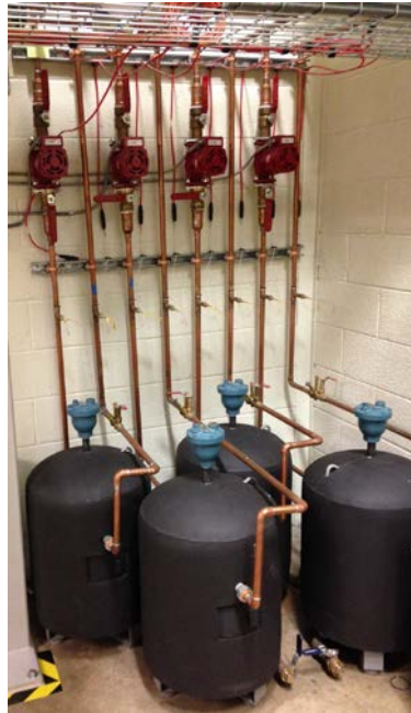
Figure 13. The black tanks hold water for the thermal mass coils in the zone simulators. Above the tanks are the red circulating pumps that move the water through the TMCs. The flow rate is determined by manually setting a valve.
