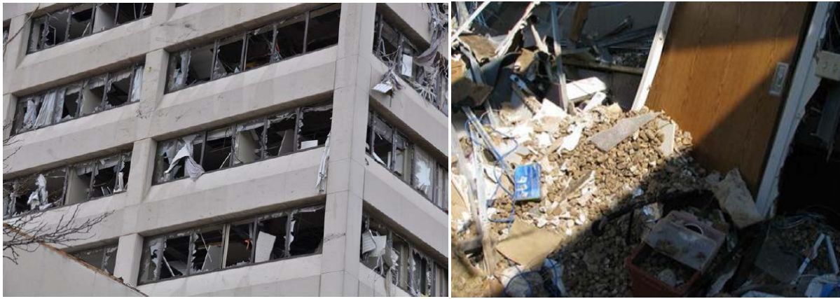
Figure 1-3 Window (left) and Interior (right 4 ) Damage to Hospital Following the Joplin, MO Tornado
