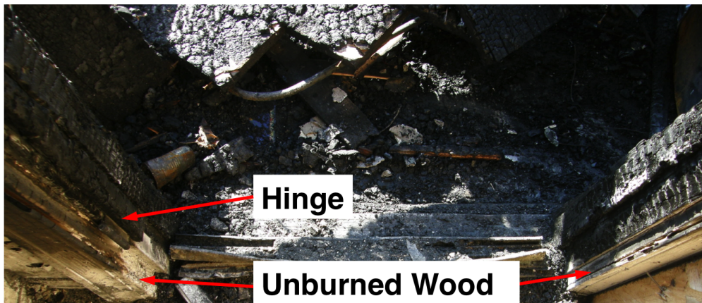
Figure 3.3: Post-incident image of the second floor porch door frame that failed taken from inside the structure looking toward the porch. Note that the hinge is still intact and there is unburned, “clean” wood along the bottom portion of the frame.
