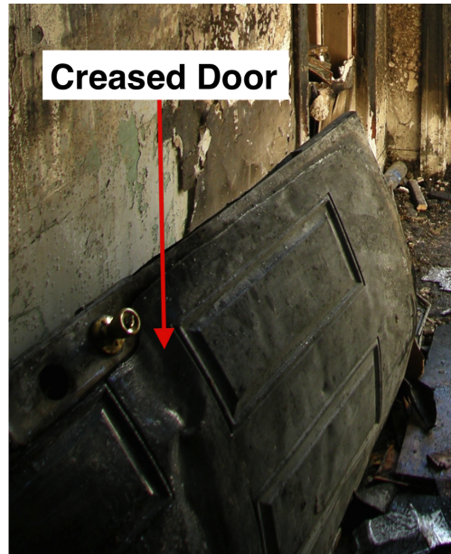
Figure 5.1: Post-fire image of interior door.
