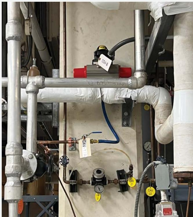
**FIGURE 2:** The newly installed CO<sub>2</sub> shutoff valve.
