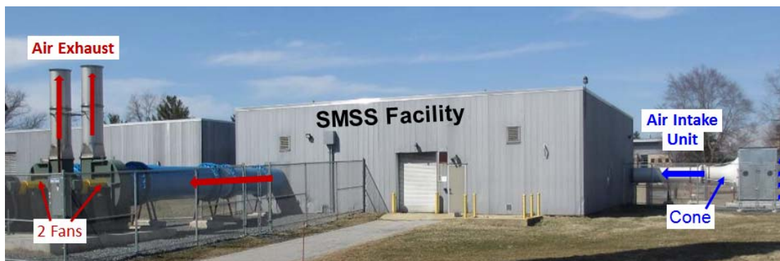
Figure 2. Scale-Model Smokestack Simulator (SMSS) showing the sections where air enters and exits the facility. RATA and CEMS performance evaluation are performed inside the building in its 1.2 m diameter Test Section.
