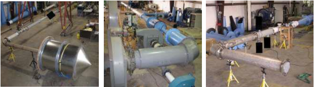
Figure 21 CEESI test facility and test piping
