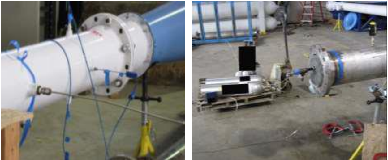
Figure 12 Tracer gas dilution installation
