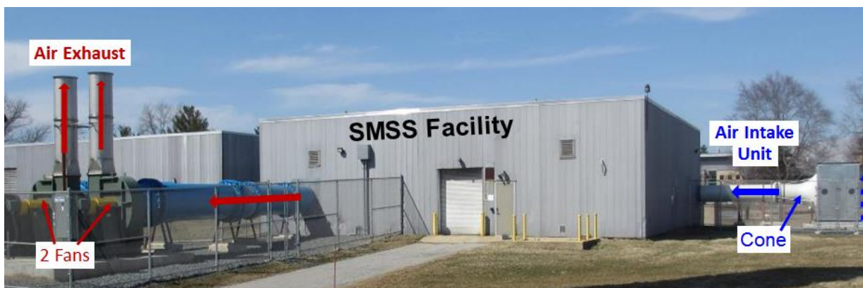
Figure 28. Photograph of the Scale-Model Smokestack Simulator (SMSS) showing the piping sections where air enters and exits the facility. RATA and CEMS performance evaluation are performed inside the building in its 1.2 m test section.
