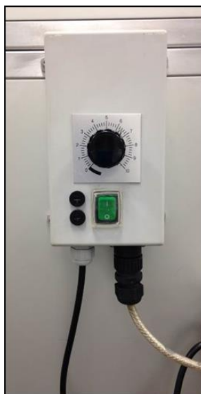
Figure 27. Thyristor control
