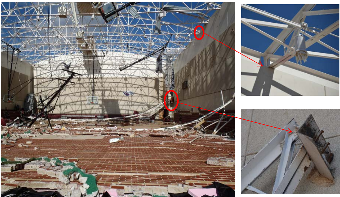
Figure 4. Example of photographic field data used in developing a failure hypothesis for the gymnasium at Joplin East Middle School. (Photo source: NIST)
