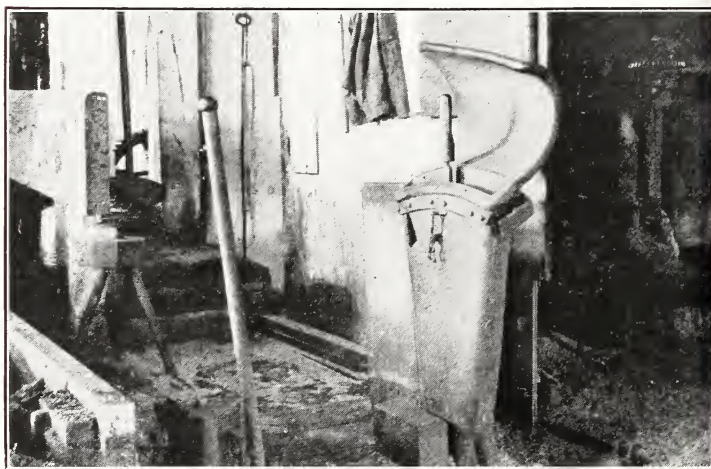
FIG. 40.—Guard for saw carriage lever. (Rule 224.)
