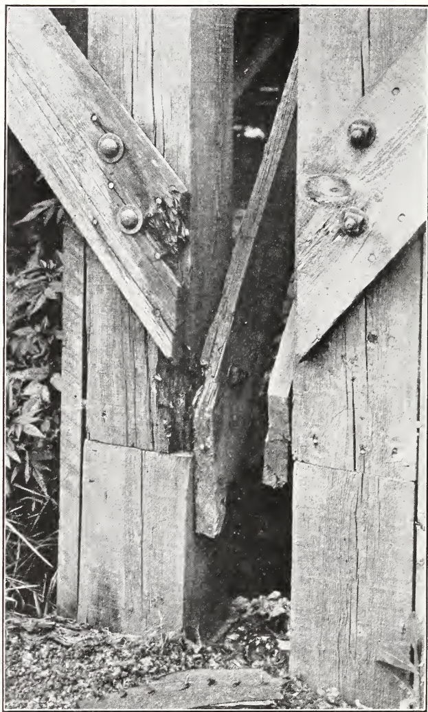
FIG. 25.—Condition of trestle footing found by inspection. (Rule 149.)
