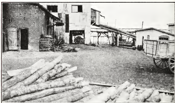
FIG. 54.—Exceptional housekeeping in mill yard; slabs carefully piled, and driveways clear of refuse. (Section 30.)
