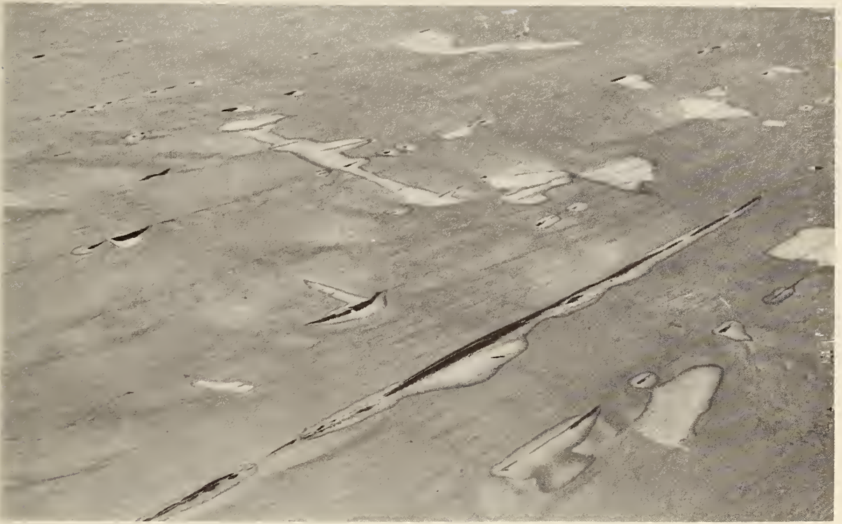
Figure 2. Membrane Wrinkling and Ridging (note water marks).
