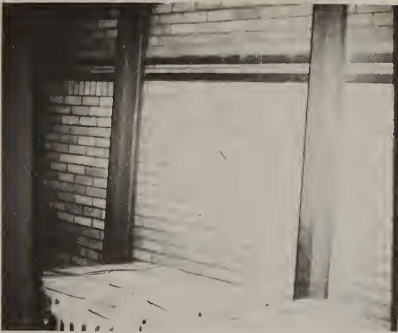
Figure 5. Outer wall of the exit of a small tunnel kiln used to fire building brick. Inner walls and ceiling constructed of refractory brick.
