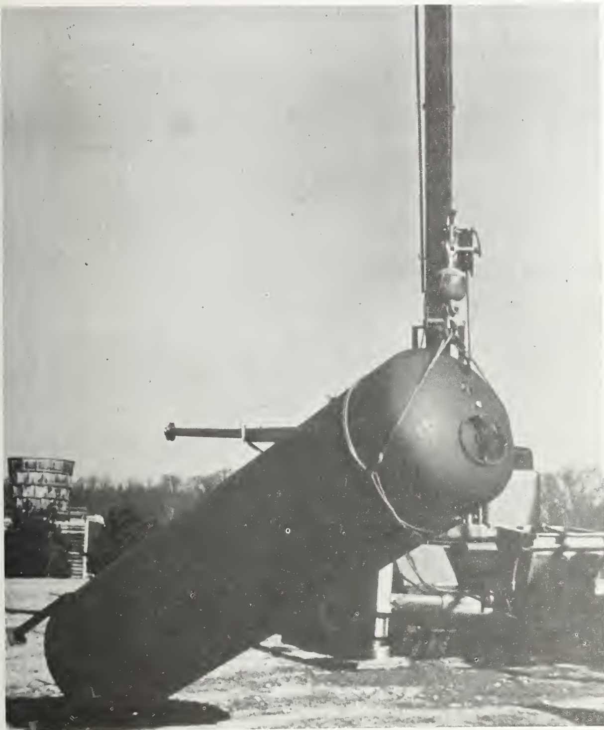
Figure 26. Moving 3.8 \text{ m}^3 (1000 gallon) storage tank into place in the NBS test house.
