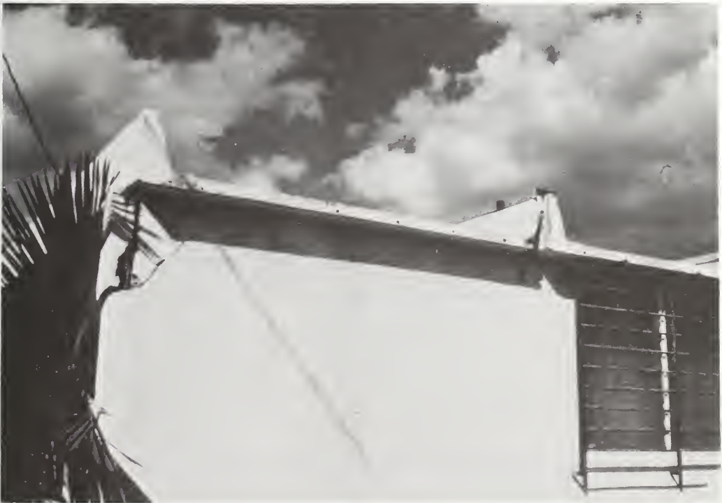
Figure 51: Bello Horizonte, walls cracked at connection of roof panels, December 30, 1972.
