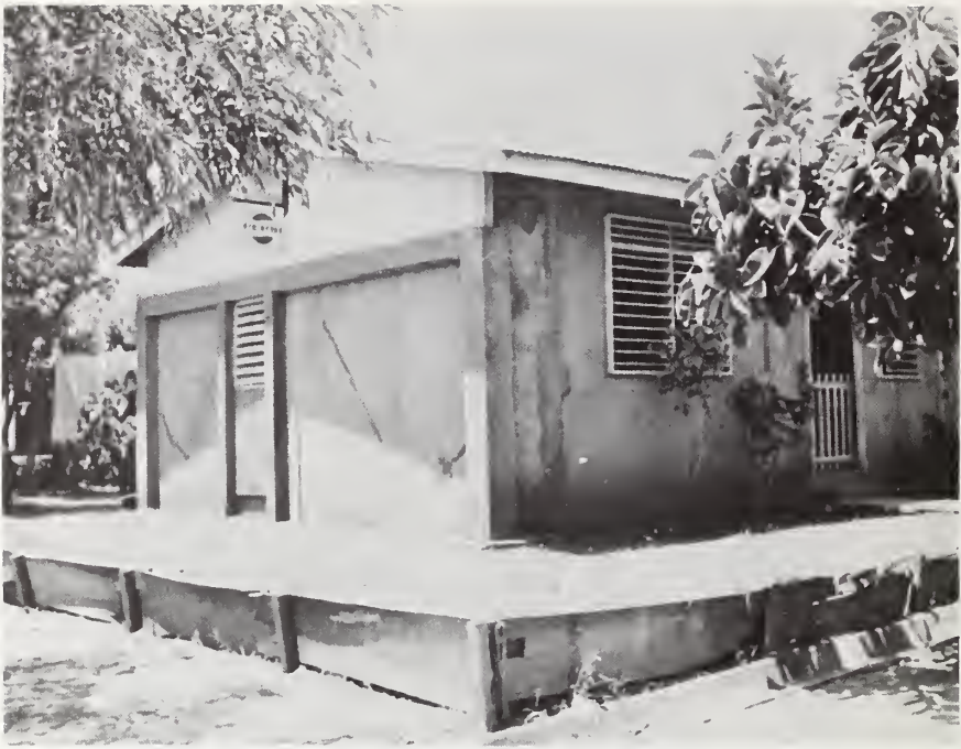
Figure 17: Colonia Maximo Jerez, less damaged frame-panel units.
