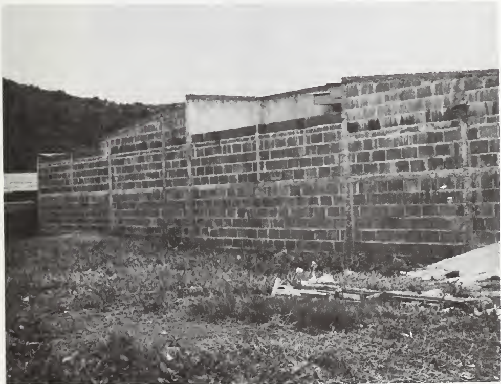
Figure 3: Las Brisas, reinforced block masonry construction.
