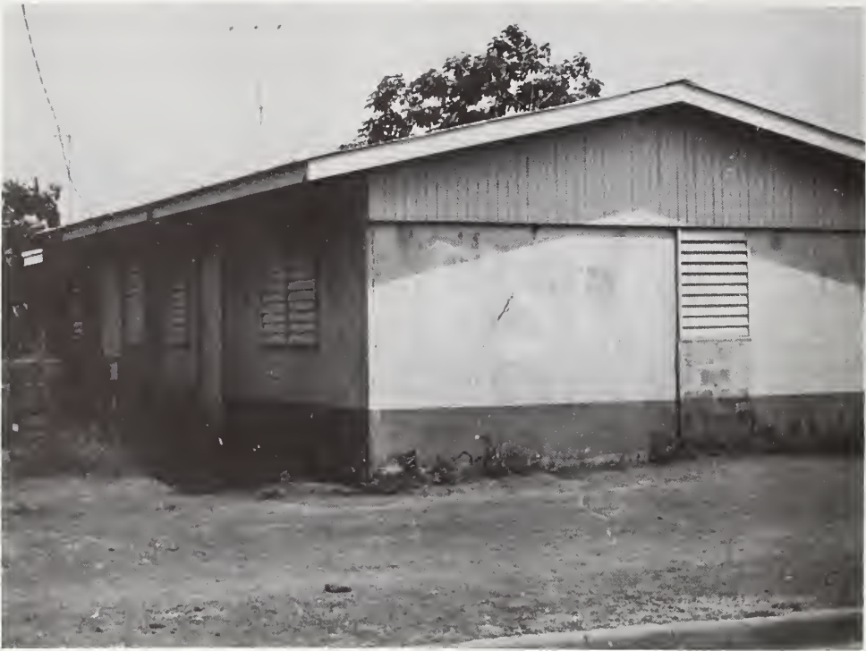
Figure 8: Colonia Francisco Morazan, cracking representative of greatest observed damage.
