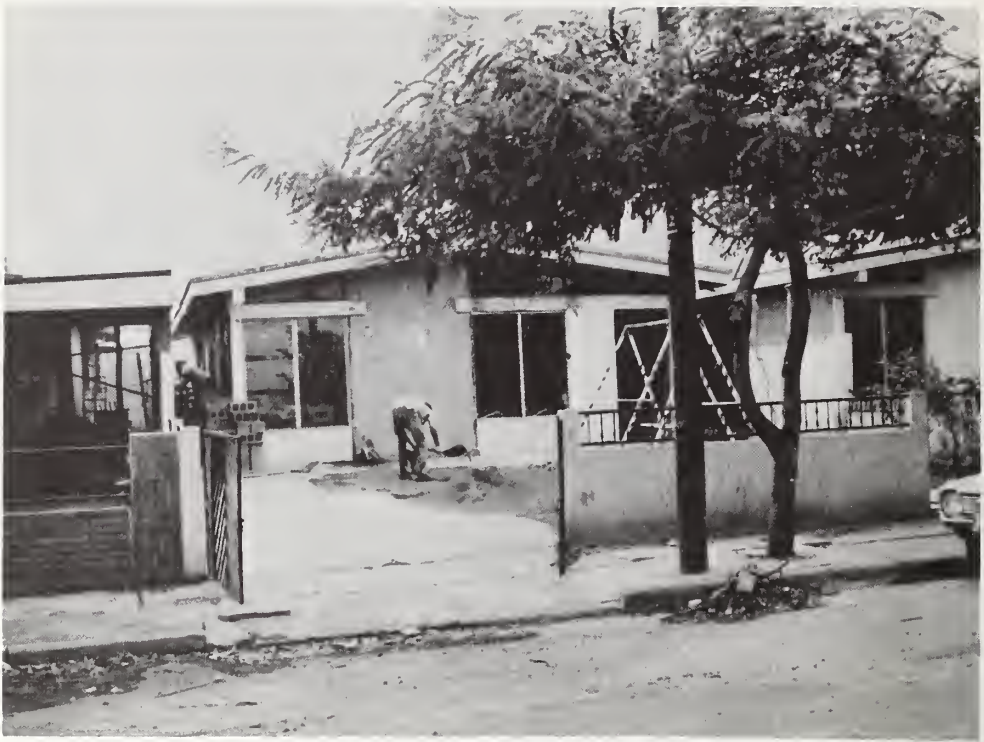
Figure 45: Ciudad Jardin, repairs of cracking and broken panels.
