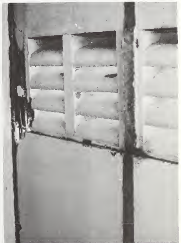
Figure 7: Las Brisas, joint where interior partition was displaced.
