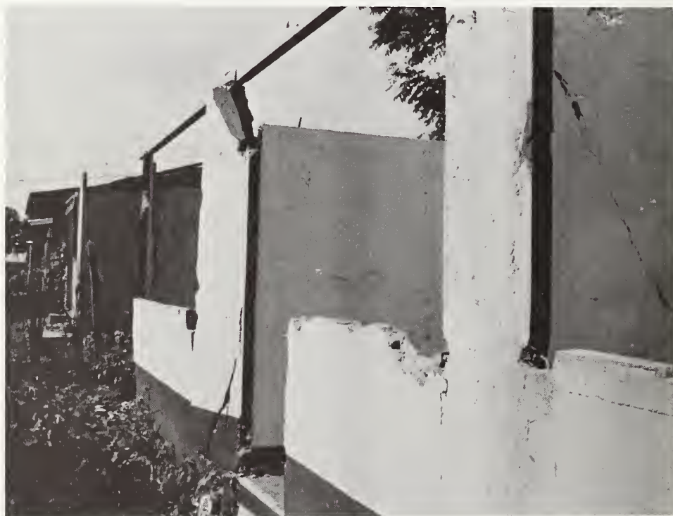
Figure 29: Colonia Nicarao, bulging of front walls.
