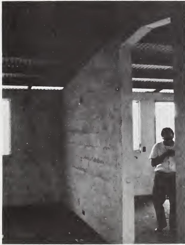
Figure 24: Colonia Luis Somoza, structural interior walls.
