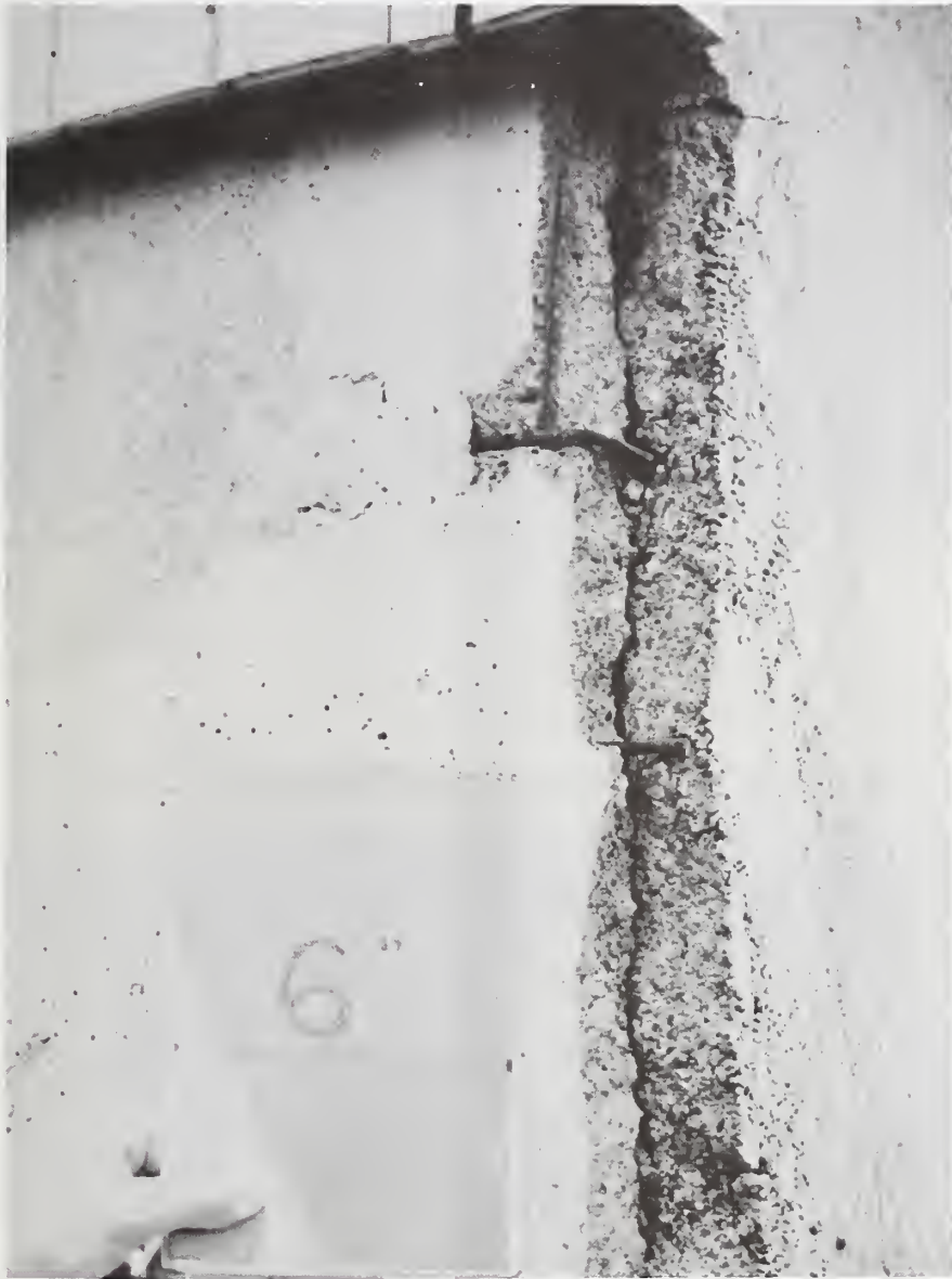
Figure 10: Colonia Francisco Morazan, opened joint at corner.
