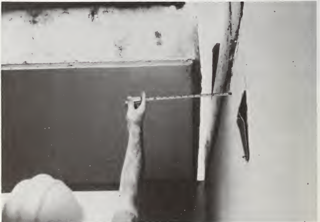
Figure 49: Bello Horizonte, lack of connection of roof to wall in duplex unit, December 30, 1972.
