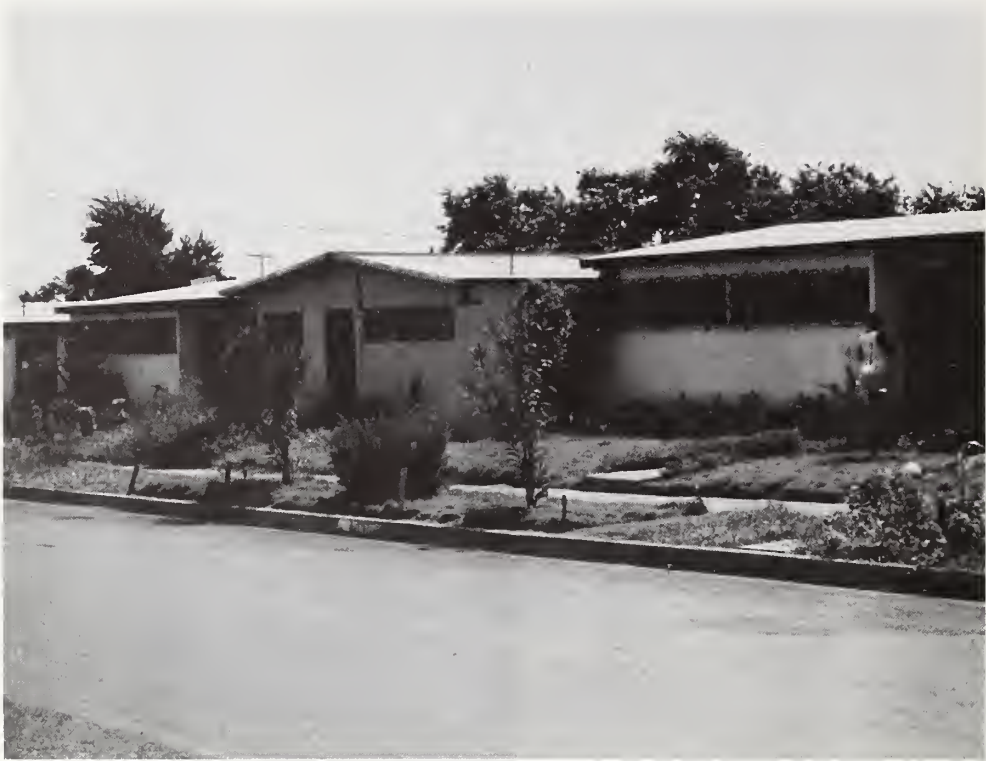
Figure 4: Las Brisas, alternate concrete panel type (failed) and reinforced masonry (in use) houses.
