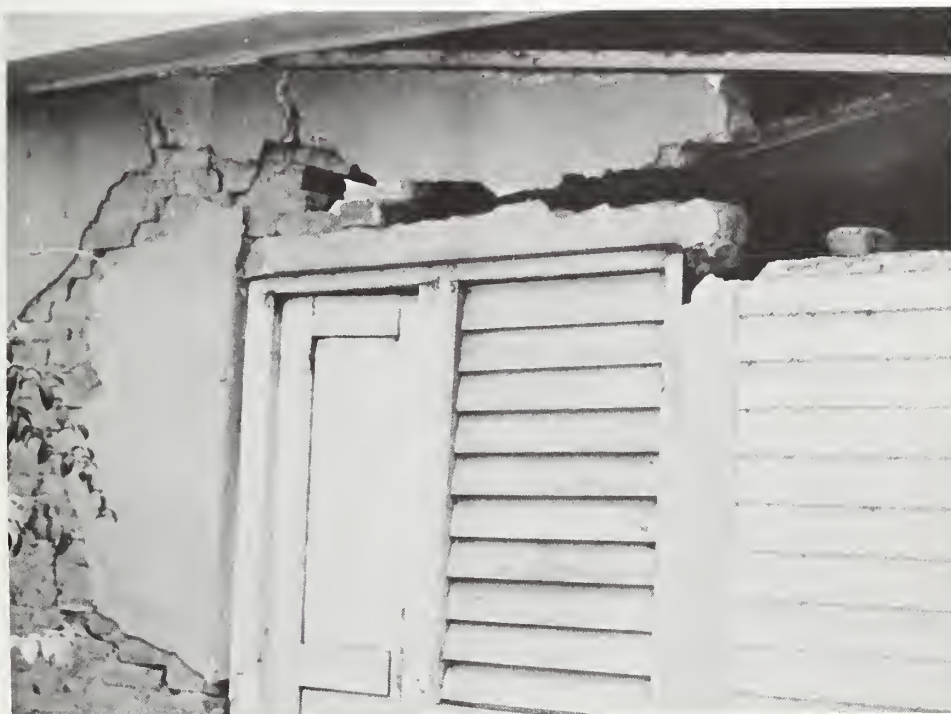
Figure 14: Barrio Monsenor Lezcano, close up of damaged masonry.
