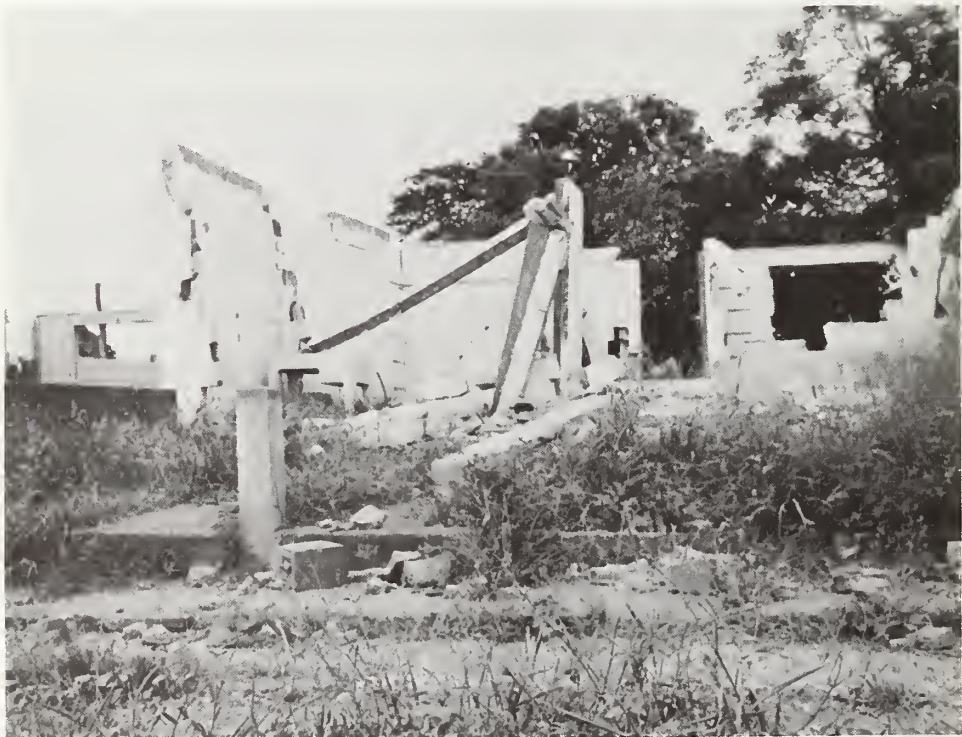
Figure 27: Barrio Ducuali, collapsed house with roof salvaged.
