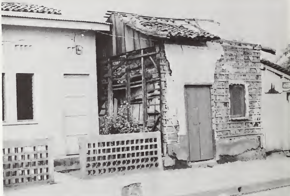
Figure 11: Barrio Monsenor Lezcano, most taquezal severely damaged or collapsed.
