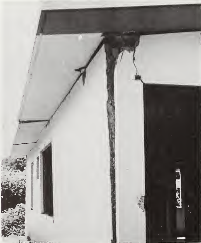
Figure 5: Las Brisas, detail of panel separations at connections.
