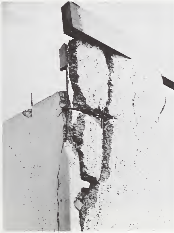
Figure 30: Colonia Nicarao, close up of corner reinforcement.
