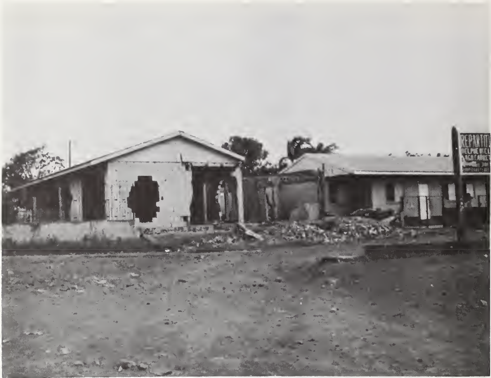
Figure 32: Colonia Nicarao, damaged grouted tile construction.
