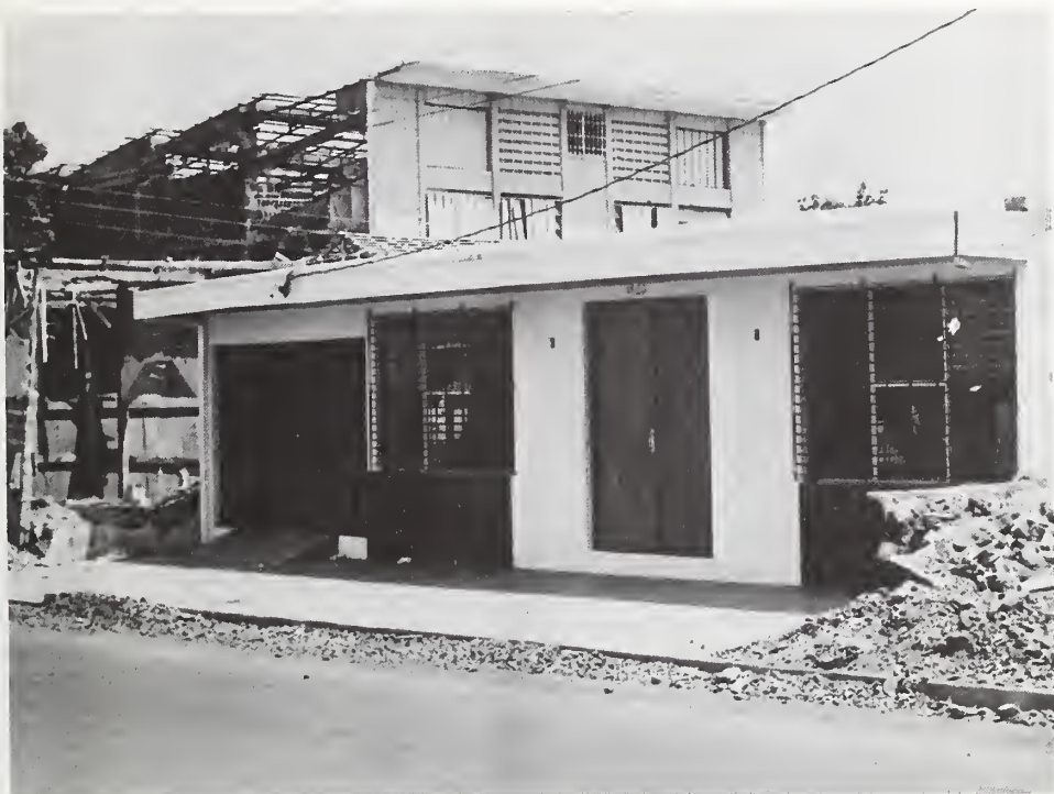
Figure 13: Barrio Monsenor Lezcano, mix of sound and collapsed buildings.
