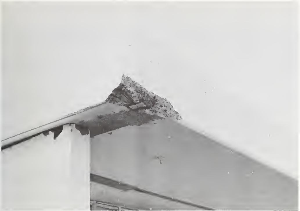
Figure 50: Bello Horizonte, weld broken and roof panel cracked at connection, December 30, 1972.
