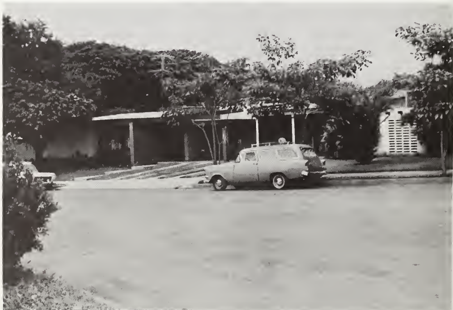
Figure 23: Los Robles, generally good condition of neighborhood.
