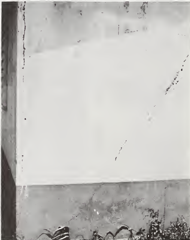
Figure 9: Colonia Francisco Morazan, cracked wall.
