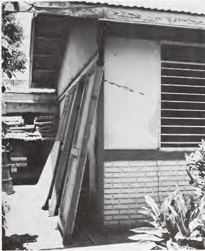
Figure 15: Colonia Managua, damage limited to cracking in poured concrete corner.
