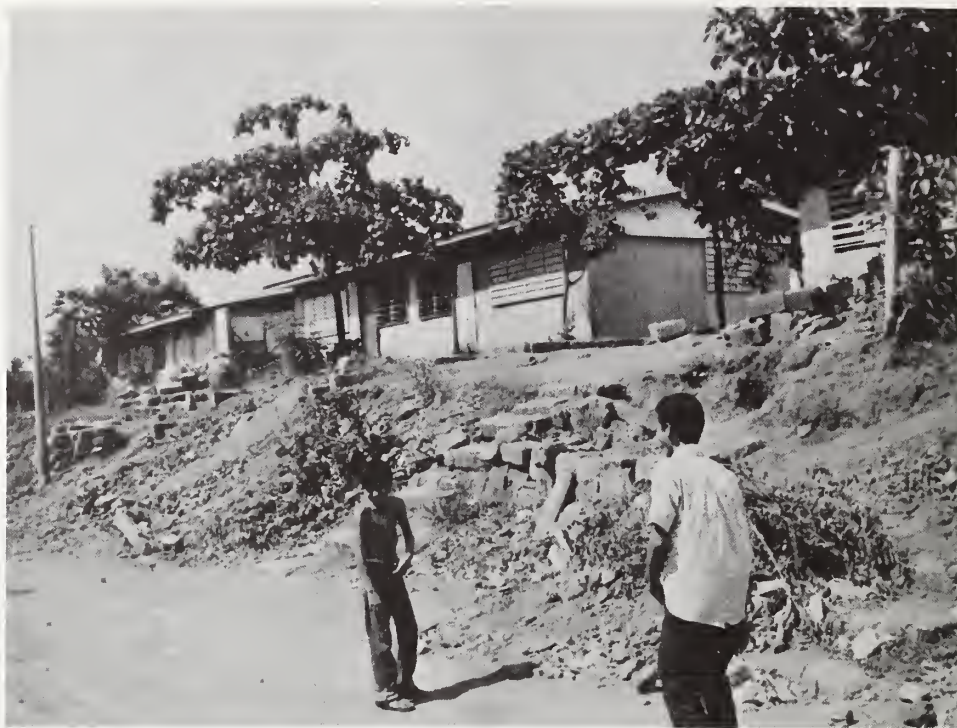
Figure 28: Colonia Nicarao, less damaged units.
