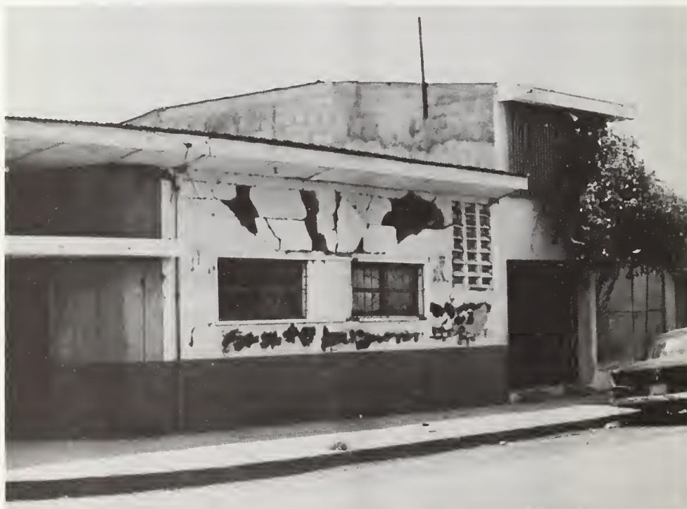
Figure 12: Barrio Monsenor Lezcano, varied performance of masonry construction.
