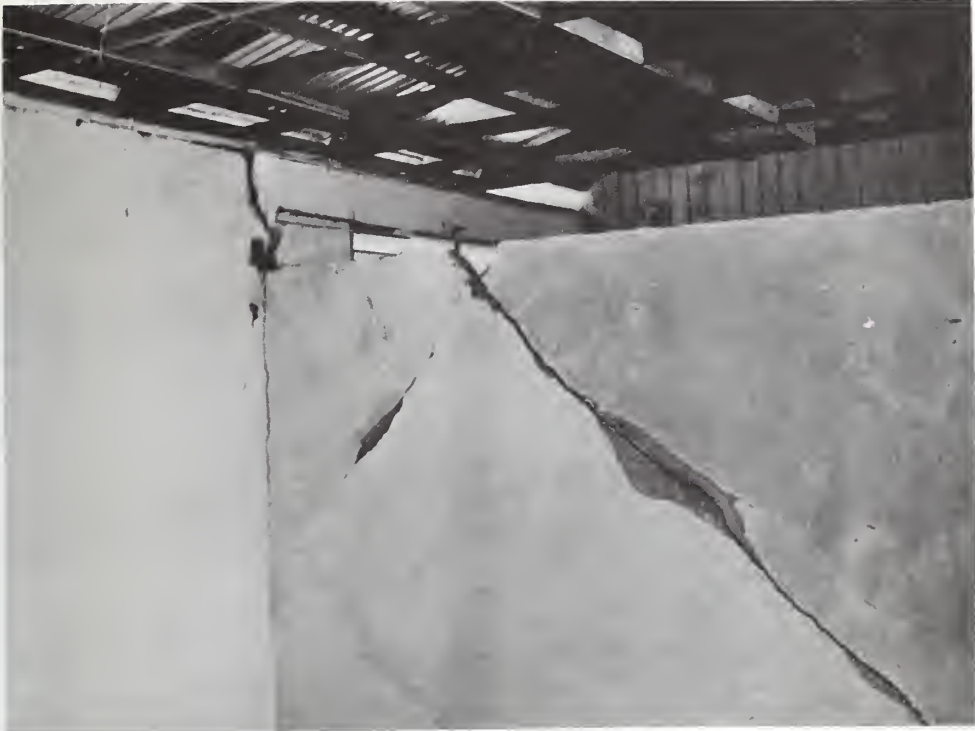
Figure 19: Colonia Maximo Jerez, damage to interior and exterior panels.
