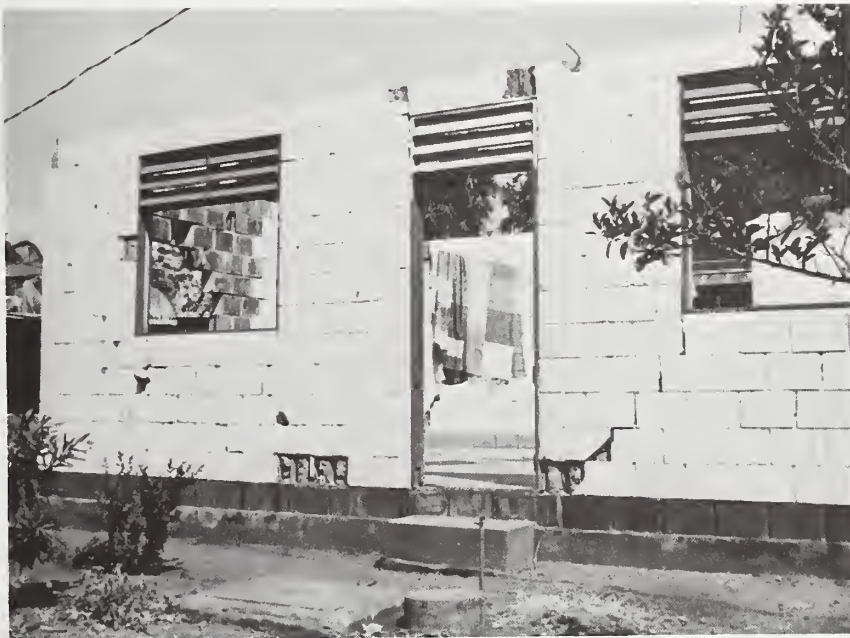
Figure 31: Colonia Nicarao, damaged grouted tile construction.
