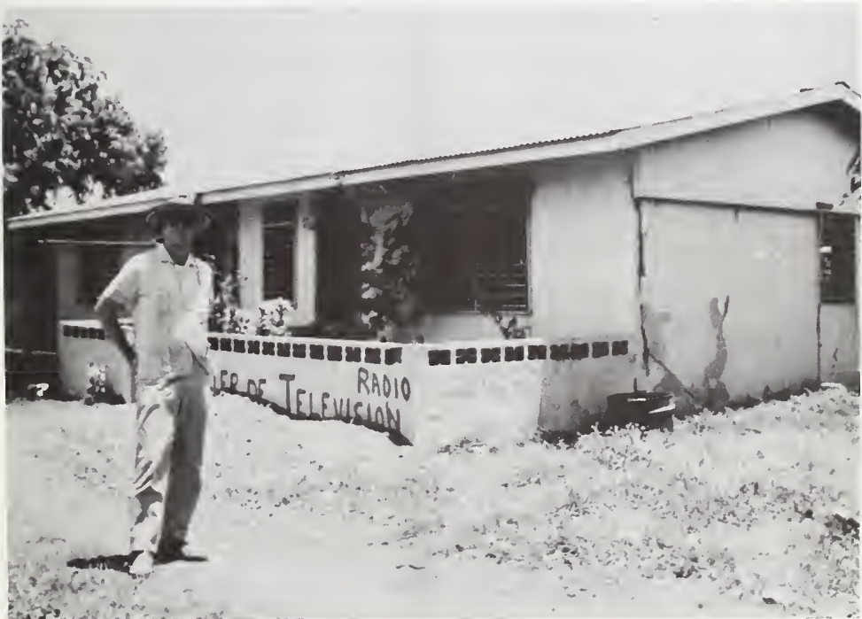
Figure 20: Colonia Maximo Jerez, unframed units showed some cracking at corners.
