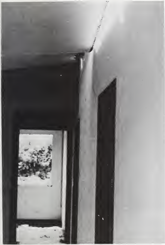
Figure 6: Las Brisas, displaced roof panel.
