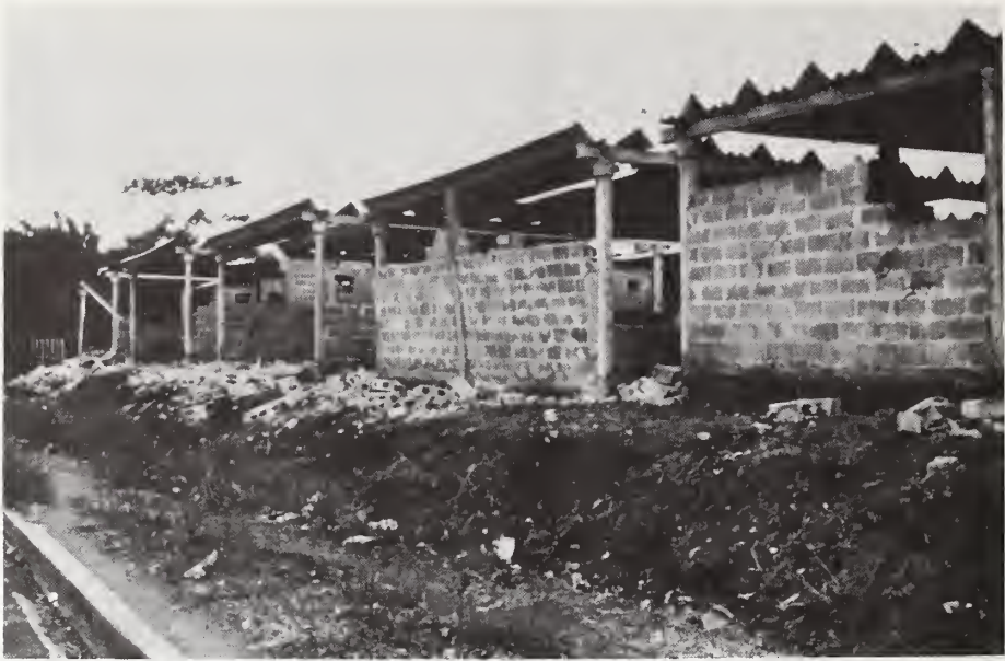
Figure 37: Viviendo de mi Hermano, frame and wall failures as seen January 3, 1973.
