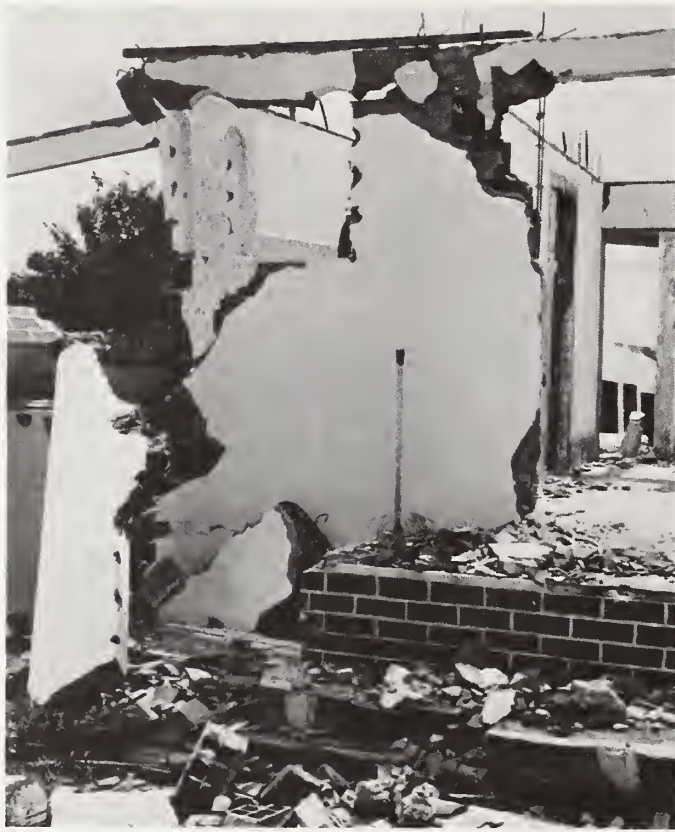
Figure 22: Los Robles, collapsed two-story house, second floor on ground.
