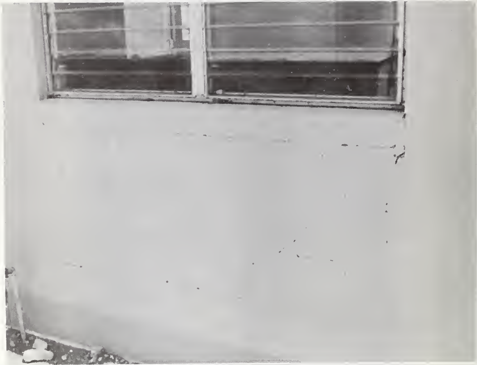
Figure 26: Colonia Luis Somoza, light cracking of blocks.
