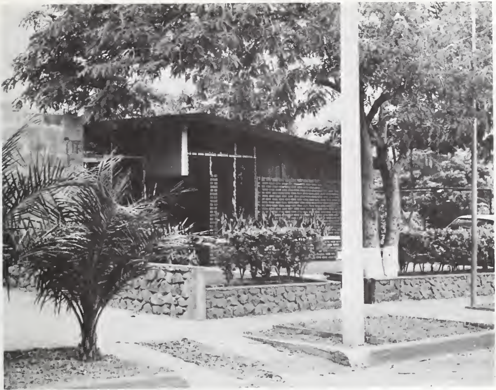
Figure 2: Las Brisas, no apparent damage to typical house.
