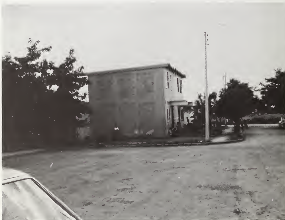
Figure 41: Proyecto Piloto, sound structural condition of two story units.
