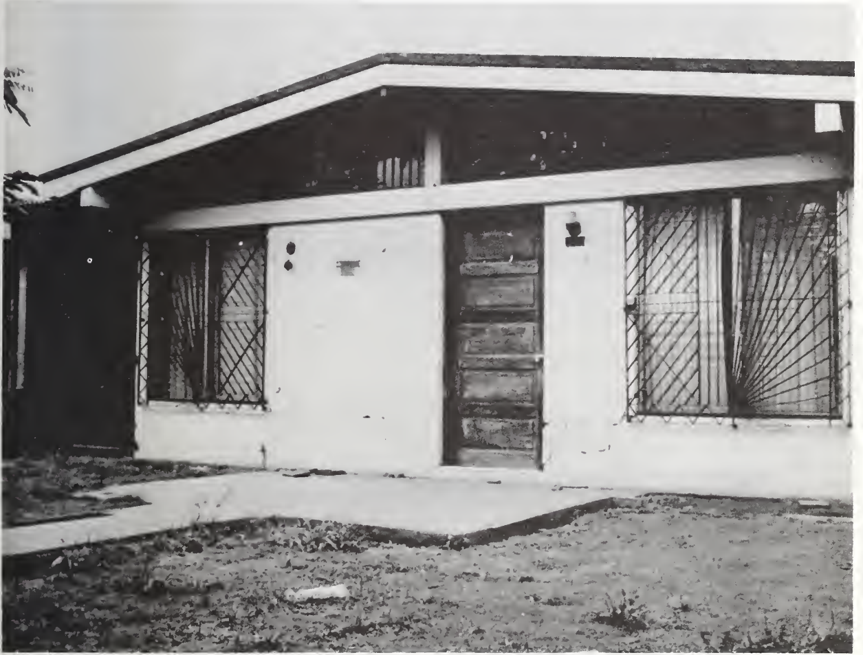
Figure 47: Ciudad Jardin, crack patterns suggesting weak mortar.
