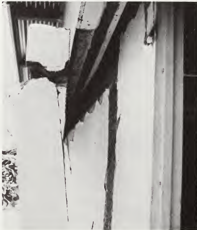
Figure 18: Colonia Maximo Jerez, separation of frame and panels.
