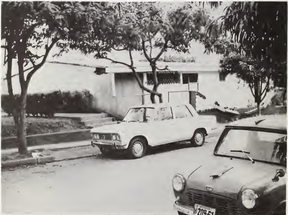
Figure 46: Ciudad Jardin, localized damage, failure of free standing walls.
